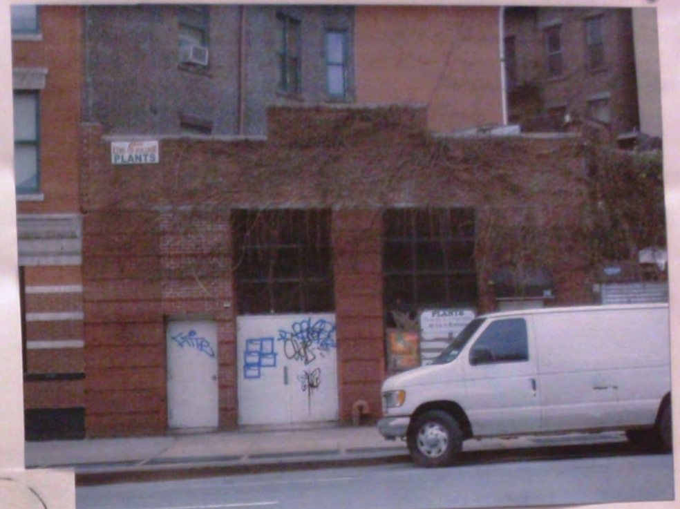
② PHOTO 1 OF PREVIOUS EXISTING CONDITIONS N.T.S.
