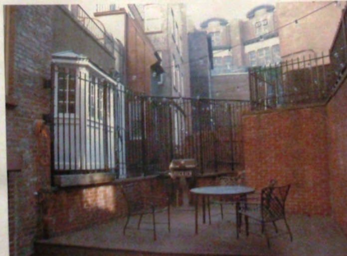
3 EXISTING ALTERATIONS IN SAME ROW -VIEW FROM 117 BEDFORD YARD
