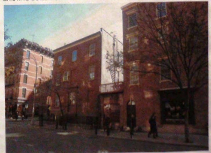
117 BEDFORD STREET -EXISTING BUILDING
