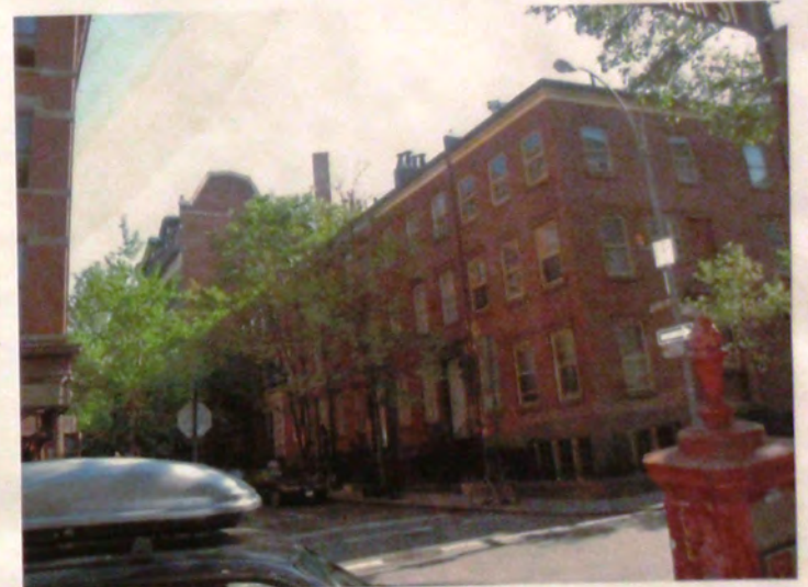
EXISTING BUILDINGS WITH 117 BEDFORD STREET
