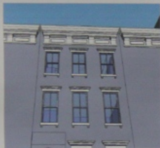
VIEW FROM WEST LEVEL AT WEST 4TH & WEST 4TH STREET
