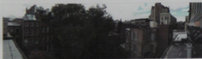
VIEW OF BUILDING FROM THE BASE OF THE ROOF ON WEST 4TH STREET
