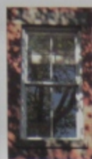
292 West 4th Street, Elevation of Second Floor Window
