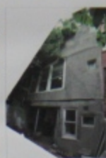
292 West 4th Street, Side Facade
