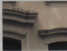
292 West 4th Street, Balcony
