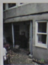
292 West 4th Street, Rear Facade
