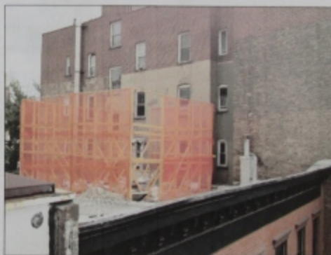
PHOTO FOR MOCK UP (TAKEN FROM ROOF OF BUILDING 245 WEST 11 STREET)
