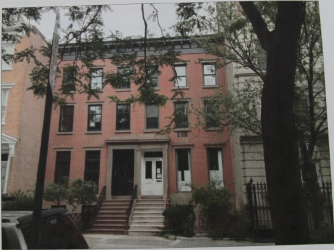
PHOTO OF EXISTING CONDITION OF BUILDING
