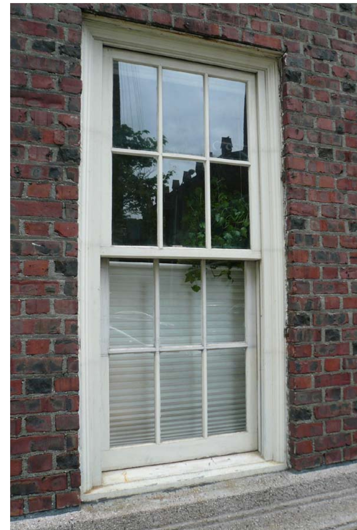
EXISTING WOOD WINDOW (TYPICAL TO 1ST-14TH FLOORS)
