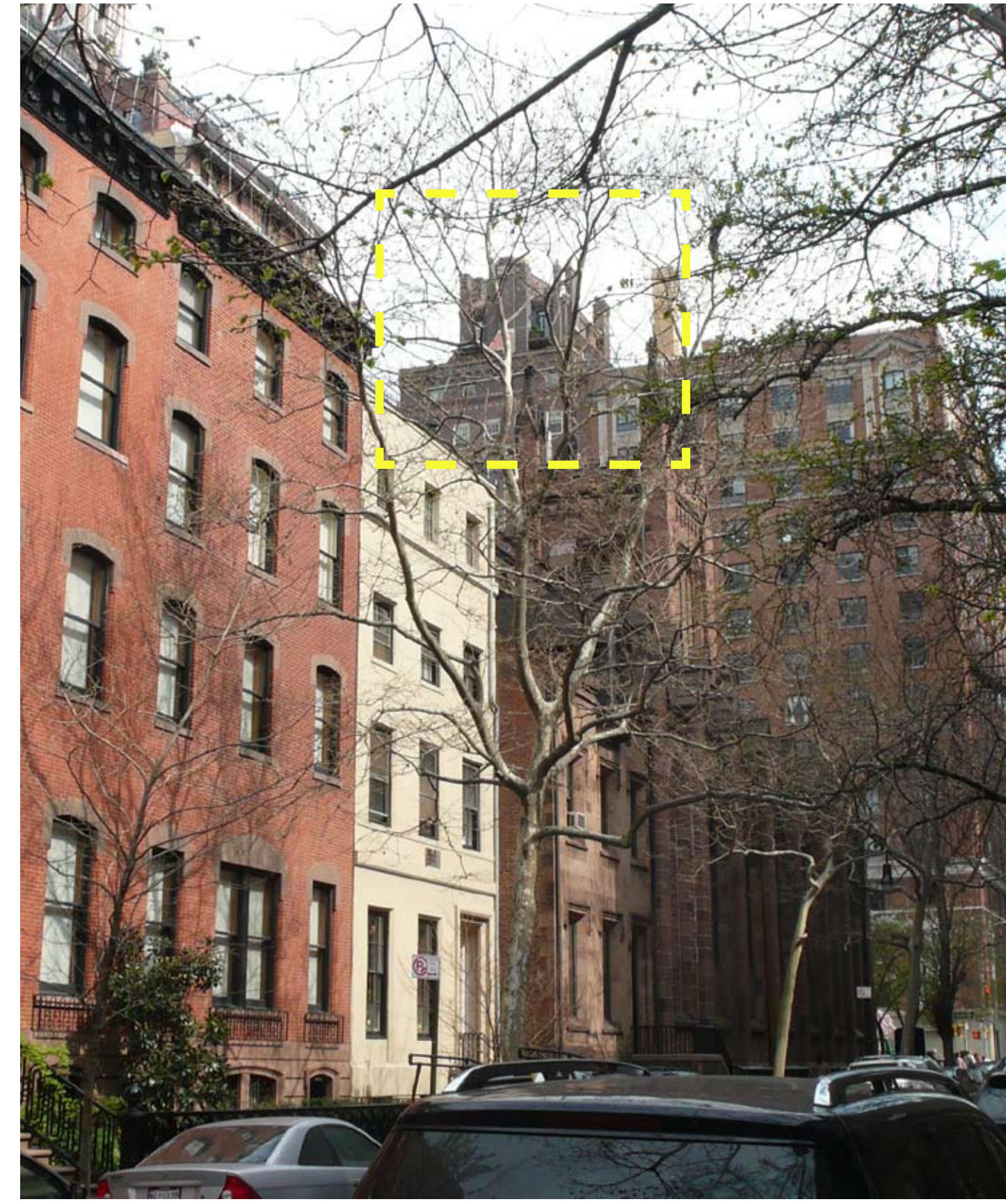
IMAGE 3 - VIEW FROM 10TH ST LOOKING EAST NEW WINDOWS PARTIALLY VISIBLE
