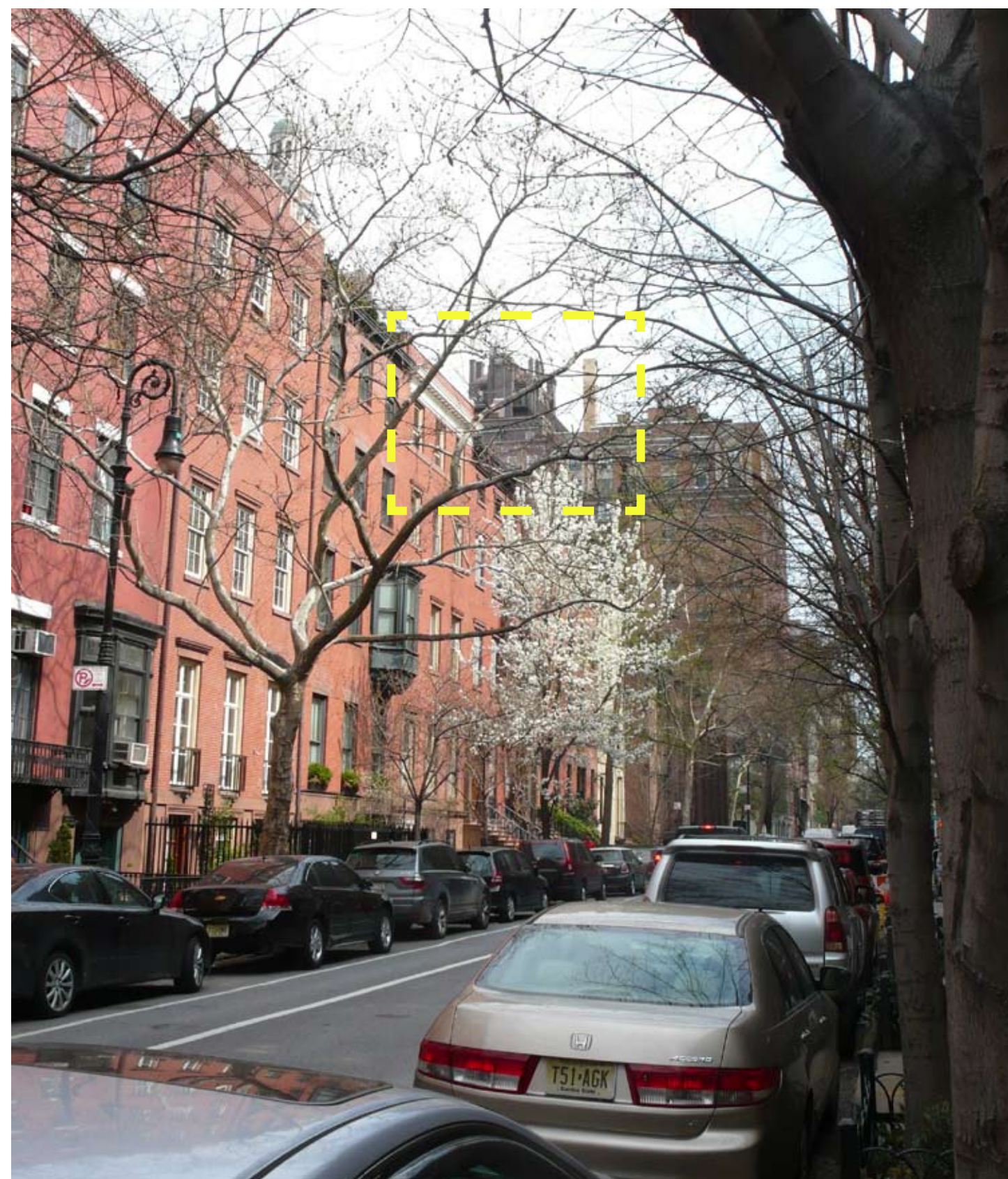
IMAGE 4 - VIEW FROM 10TH ST LOOKING EAST NEW WINDOWS PARTIALLY VISIBLE
