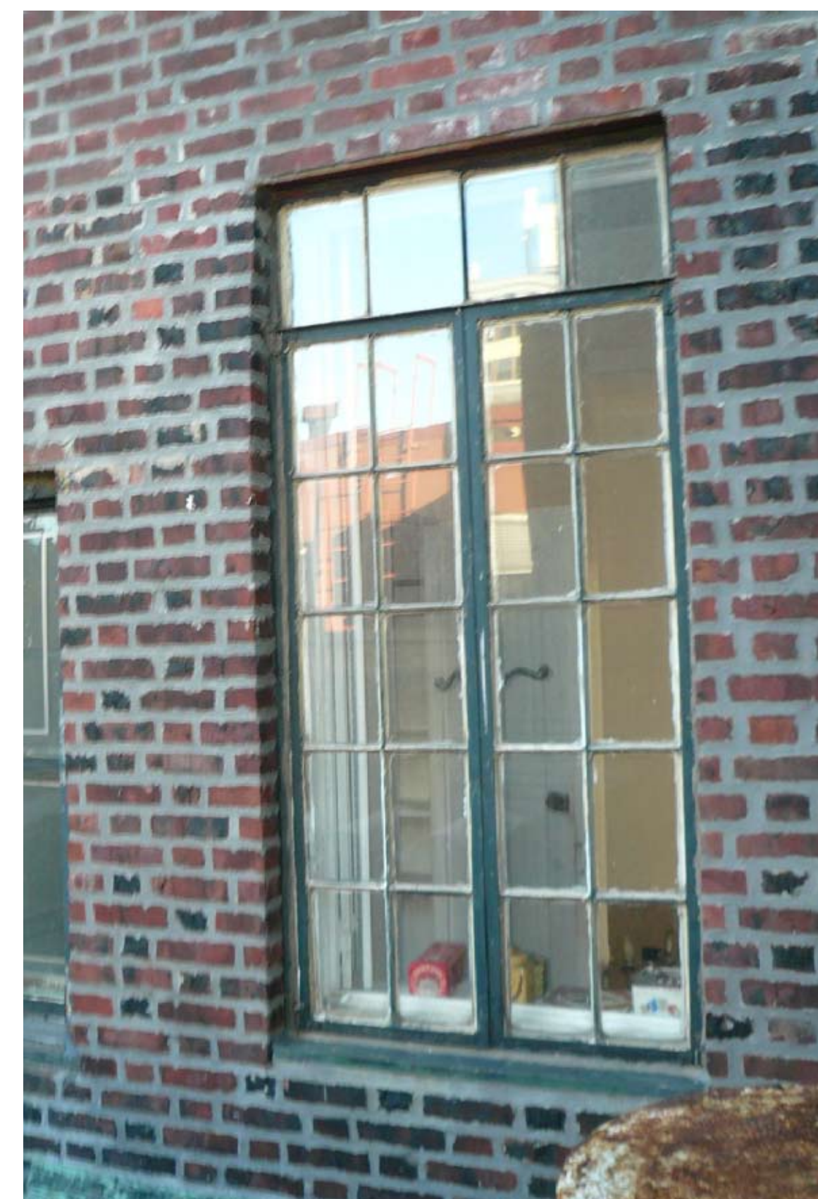
EXISTING STEEL WINDOW (TYPICAL TO 15TH FLOOR)
