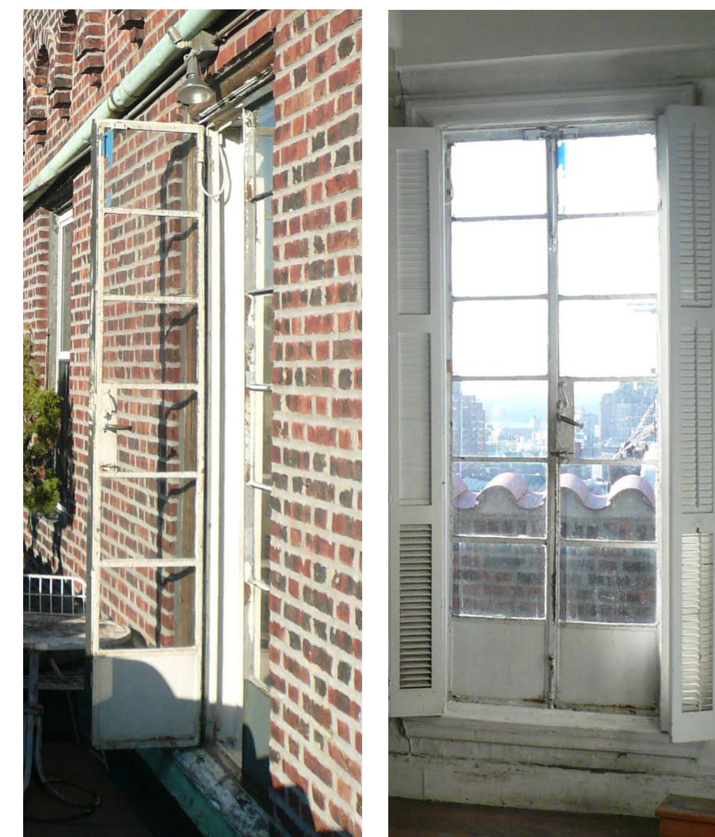
EXISTING TERRACE DOOR AT 15TH FLOOR (EXTERIOR AND INTERIOR VIEWS SHOWN)
