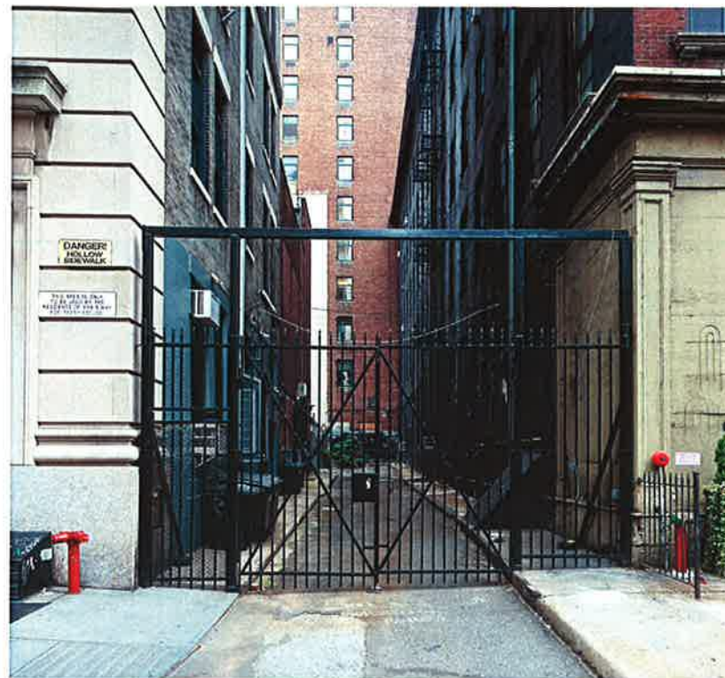
5 1034_GATE 3B_EXISTING GATE
