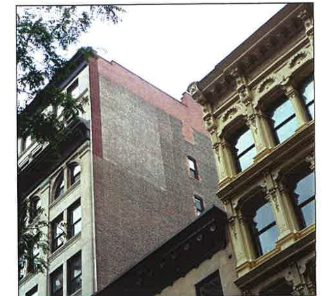
7 EXPOSED LOT LINE WALLS & DIFFERENT HGT BUILDINGS ARE TYPICAL TO DISTRICT
