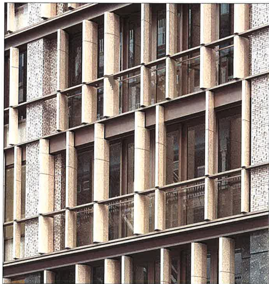
② DETAIL VIEW OF FACADE FINS
