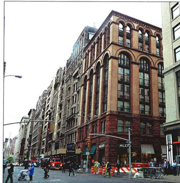
LACK OF SETBACKS ALONG B'WAY
