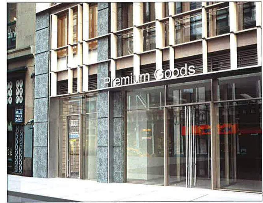
4 VIEW OF ENTRANCE
