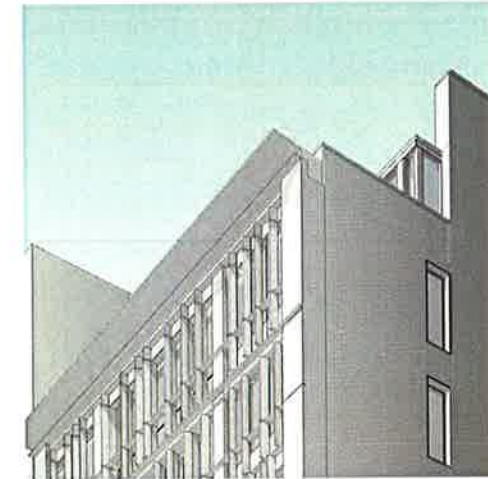
2 VIEW OF CORNICE FROM BROADWAY
