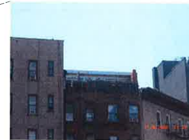
7 13 7TH AVENUE VISIBLE ADDITION AT ROOFTOP OF ALUMINUM AND GLASS ABOVE EXISTING MASONRY.
