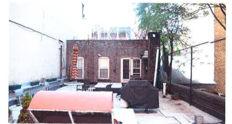
G17 VIEW TOWARDS BACK OF 129 CHARLES STREET
