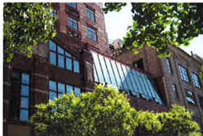
19 132 PERRY STREET MODERN SLOPED WINDOW INSTALLED ABOVE TERMINATION OF MASONRY FACADE.
