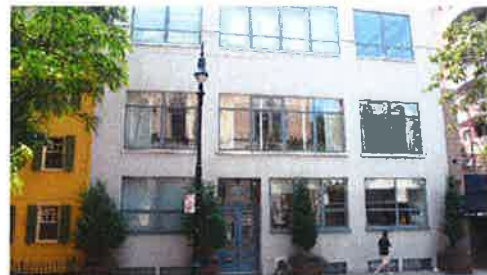
18 134-136 CHARLES STREET THIRD STORY ADDITION ADDED IN 1989 ABOVE EX'G HORIZONTAL STONE PARAPET. NEW WINDOWS AND BRICK FLUSH TO EXISTING FACADE FACE.
