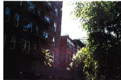
22 19 BETHUNE STREET SLOPED WINDOW OF NEW ADDITION VISIBLE FROM STREET. DETAIL OF WINDOW CREATES "STYLIZED" CORNICE.
