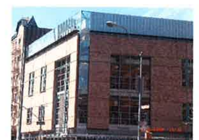
6 97 GREENWICH AVENUE NEW CONSTRUCTION, WITH CLEAR DIFFERENTIATION BETWEEN METAL CLADDING AND BRICK MASONRY DEFINED BY A STYLIZED CORNICE.
