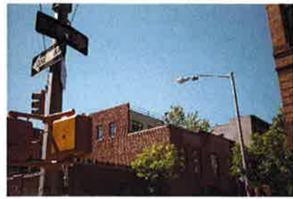
23 790 GREENWICH STREET ROOFTOP ADDITION WHICH CONTINUES THE USE OF BRICK FROM THE ORIGINAL PARTY WALL BELOW.
