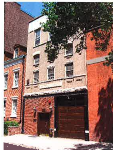
P9 VIEW TO SITE LOOKING NORTHWEST ON CHARLES STREET
