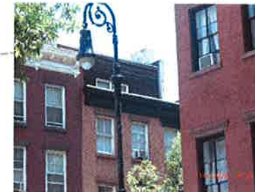
9 241 W 4TH STREET VISIBLE ADDITION IN CORRUGATED METAL SIDING ABOVE EX'G CORNICE.
