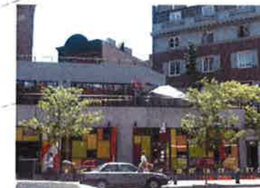
8 87 7TH AVENUE SOUTH NEW CONSTRUCTION WITH VISIBLE CONTEMPORARY SETBACK AT ROOF.
