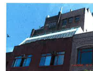
5 221 W 13TH STREET SLOPED WINDOW OF NEW ADDITION VISIBLE FROM STREET.
