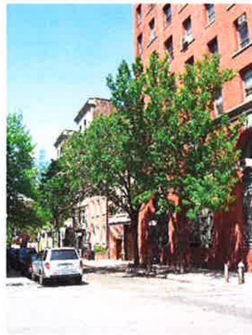
P7 VIEW FROM THE CORNER OF CHARLES STREET AND GREENWICH STREET LOOKING NORTHWEST
