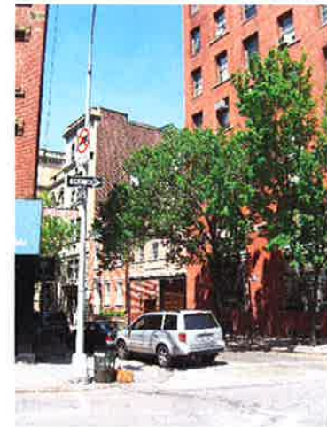
P8 VIEW FROM THE CORNER OF CHARLES STREET AND GREENWICH STREET LOOKING WEST
