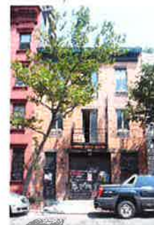
16 271 W 10TH STREET BUILDING WAS ORIGINALLY USED AS A HORSE STABLE.
