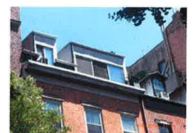
12 61 MORTON STREET VISIBLE DORMER ADDITIONS ABOVE EX'G CORNICE.
