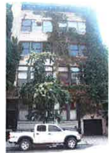
20 695-697 WASHINGTON STREET SEAMLESS ADDITION OF 2 STORIES ABOVE EXISTING FACADE COMPLETED IN 1980.
