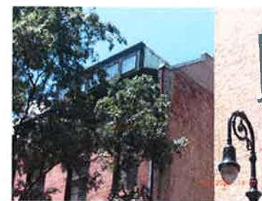
4 9 BANK STREET VISIBLE NEW DORMER AT TOWNHOUSE.
