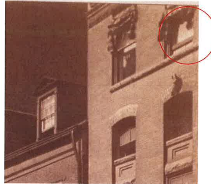
2 OVER 2 WINDOWS OF 129 CHARLES STREET, CA. 1928 (FROM NYPL DIGITAL GALLERY, ITEM 718626F)
