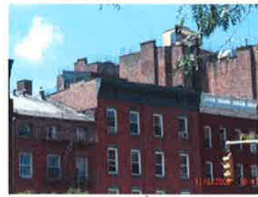
1 603 HUDSON STREET SLOPED SOLARIUM ADDITION TO ROOFTOP.
