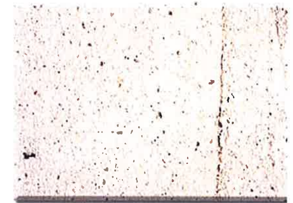
MATERIAL POURED IN PLACE CONCRETE LOCATION REAR (NORTH) ELEVATION ITEM EXTERIOR WALLS AT REAR, GROUND FLOOR PLINTH, CUSTOM PAVERS AT TERRACES
