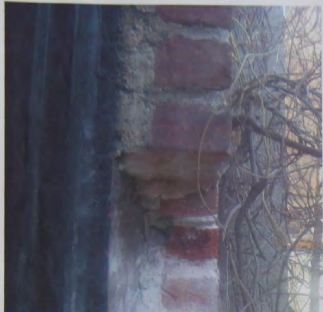
PROBE REVEALING ORIGINAL BRICK FACADE
