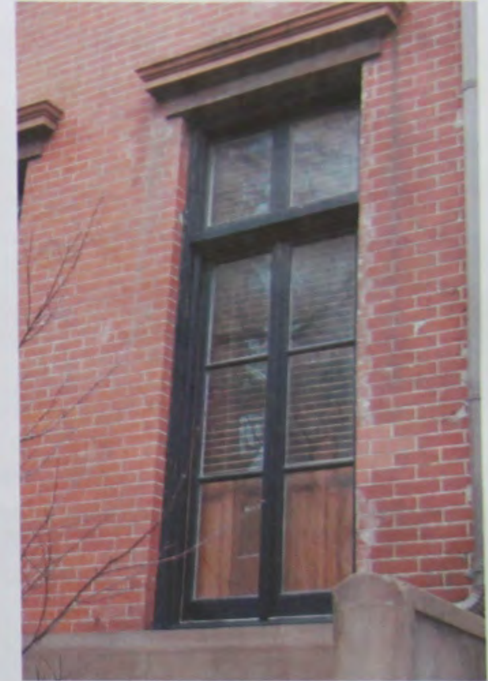
117 WEST 12 STREET PARLOR FLOOR WINDOW
