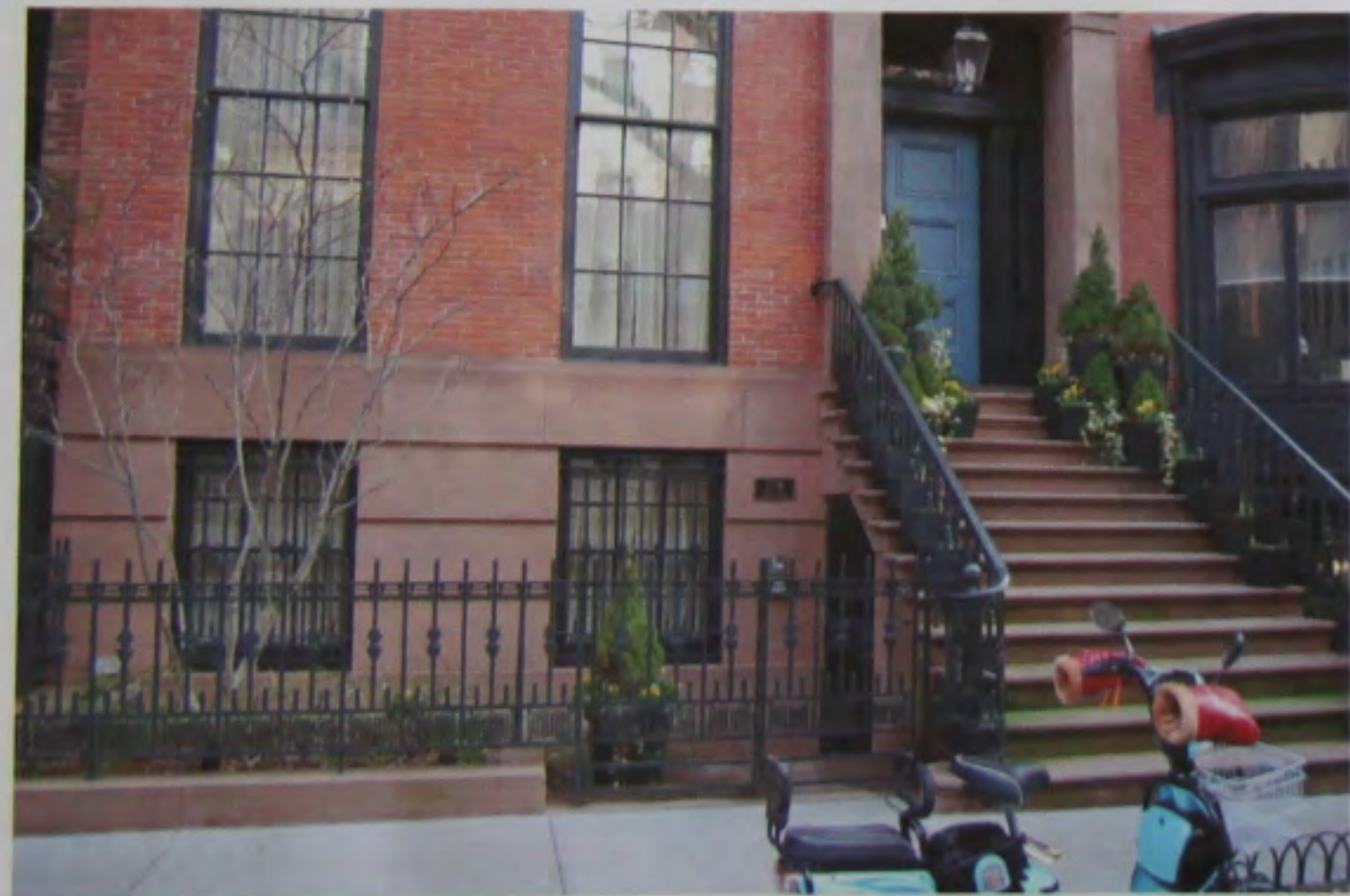
10 WEST 10 STREET IRON WORK
