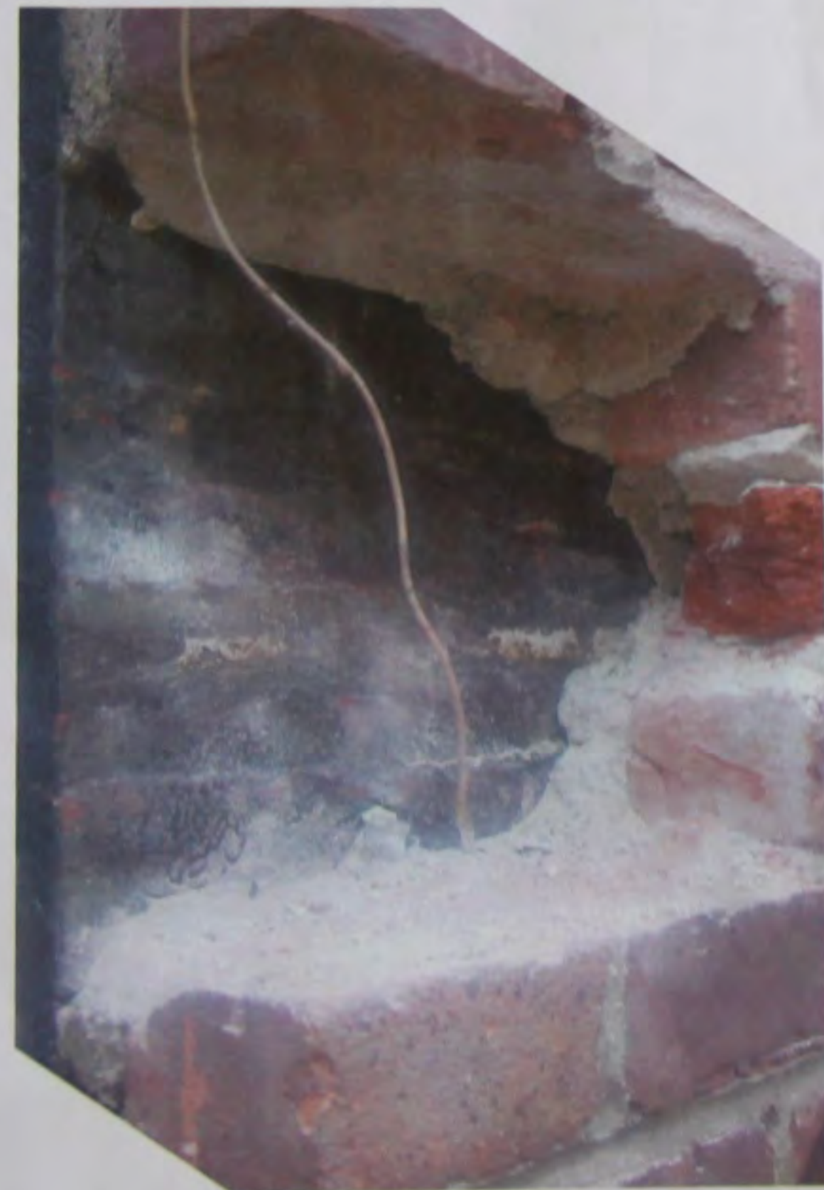
ORIGINAL BRICK FACADE BEHIND NEWER VENEER MASONRY
