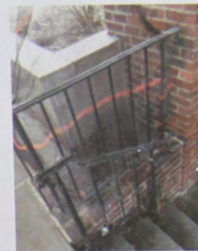
LEFT HAND RAIL ENTRANCE WAY
