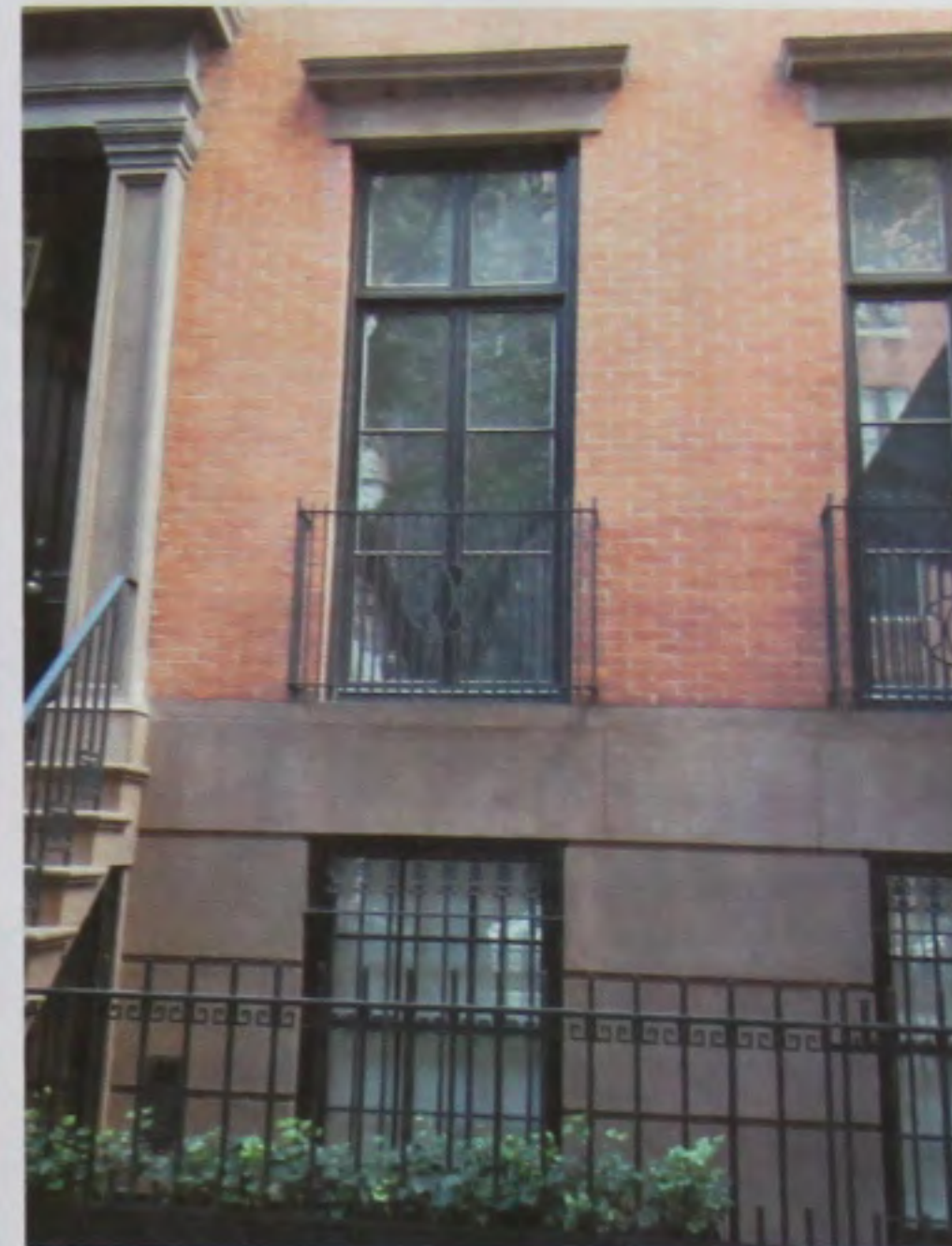
6 EAST 10 STREET PARLOR FLOOR WINDOWS RUSTICATION AT BASE
