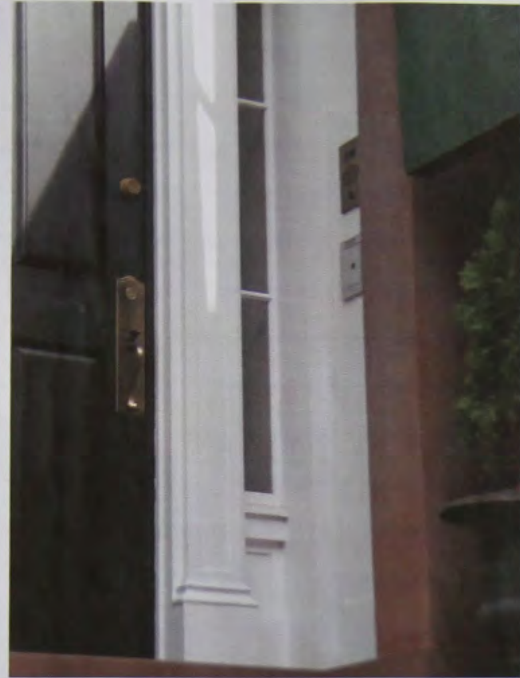
19 WEST 12 STREET ENTRANCE DOOR SIDELIGHT
