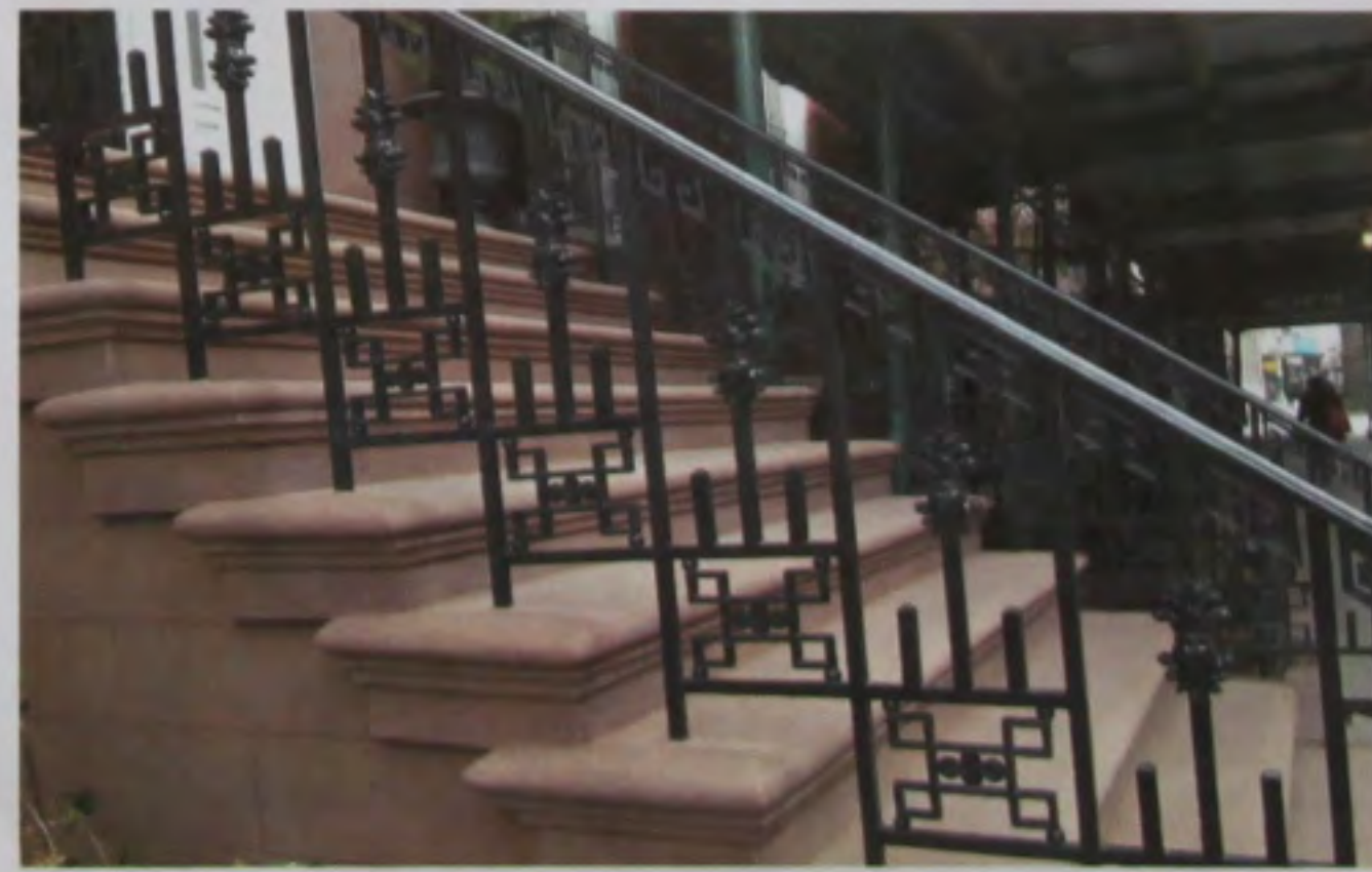
19 WEST 12 STREET IRON WORK AT RAILING
