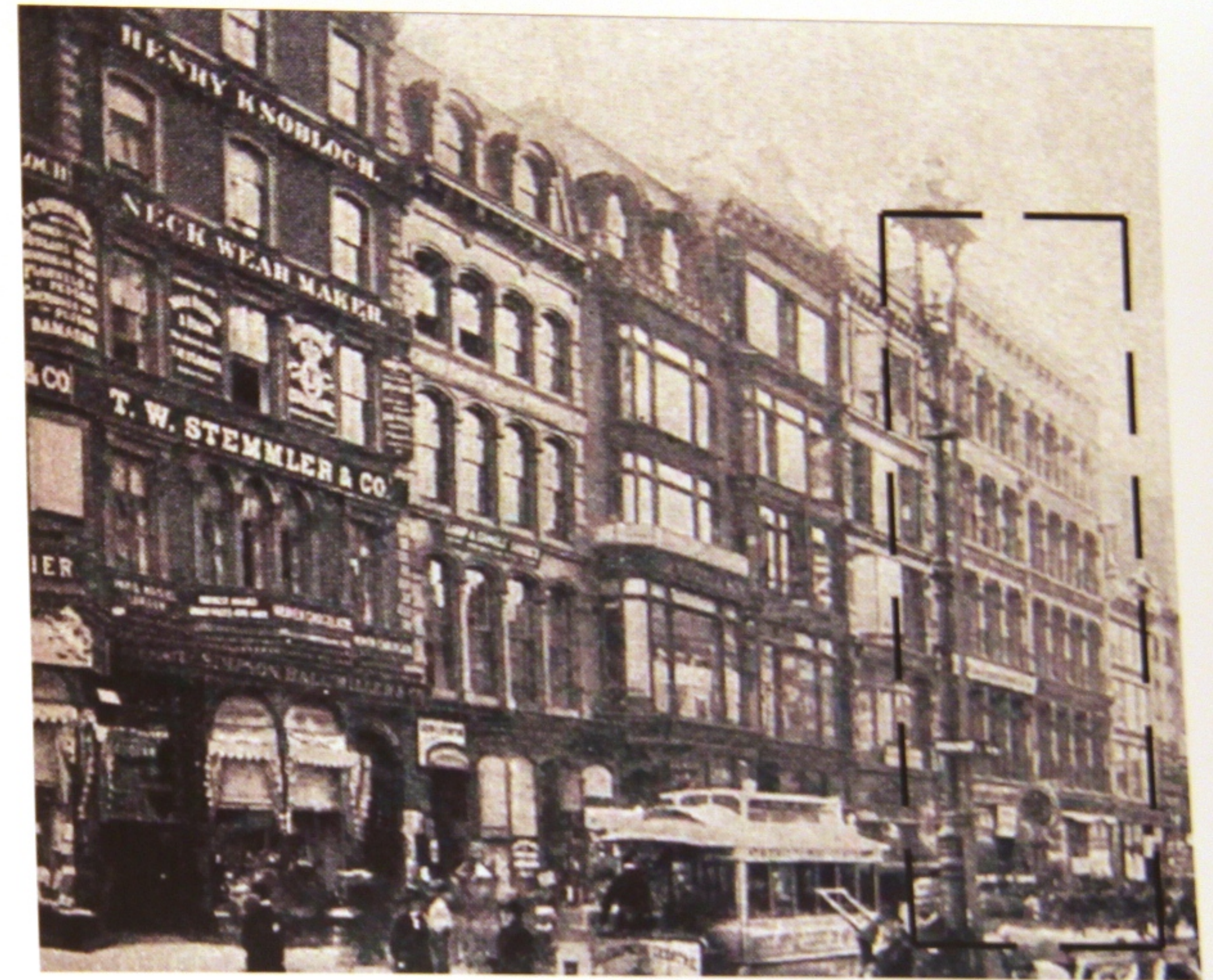
View from NW side of E 14th Street (1895)
