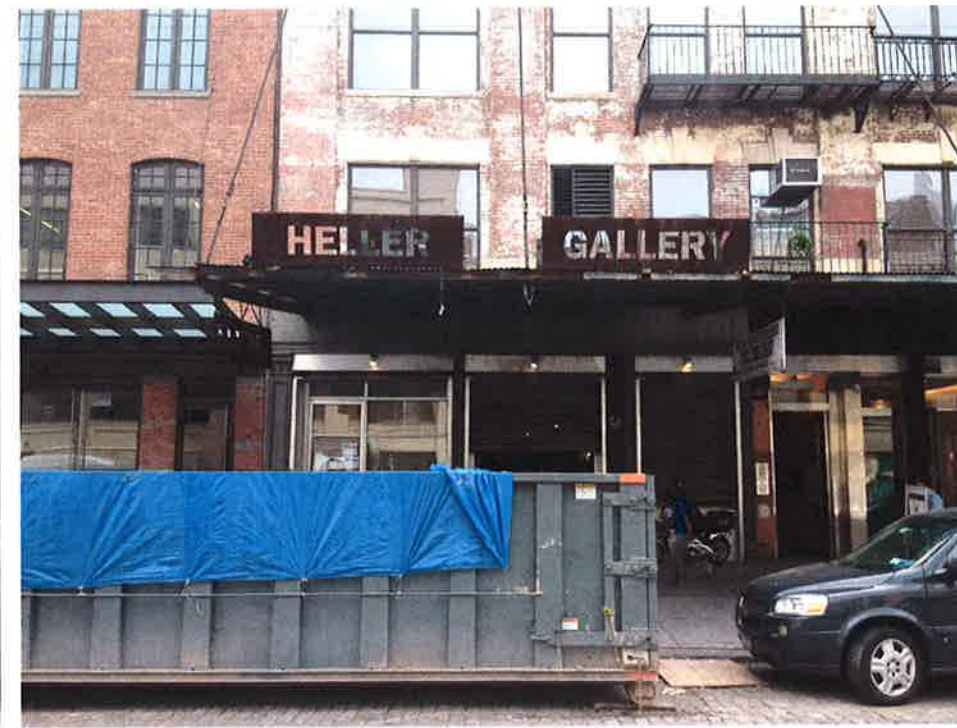
2 EXISTING FACADE – 420 W 14TH ST SCALE: NA
