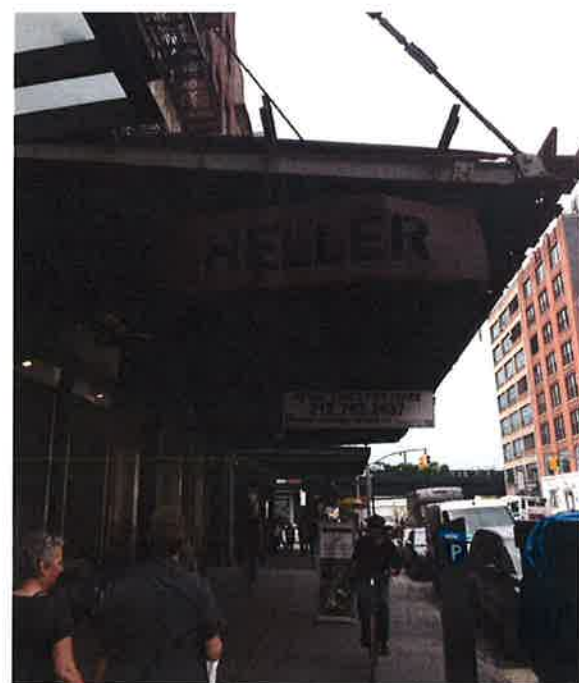
5 EXISTING FACADE – 420 W 14TH ST SCALE: NA
