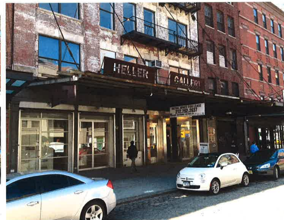
1 EXISTING FACADE – W 14TH ST SCALE: NA
