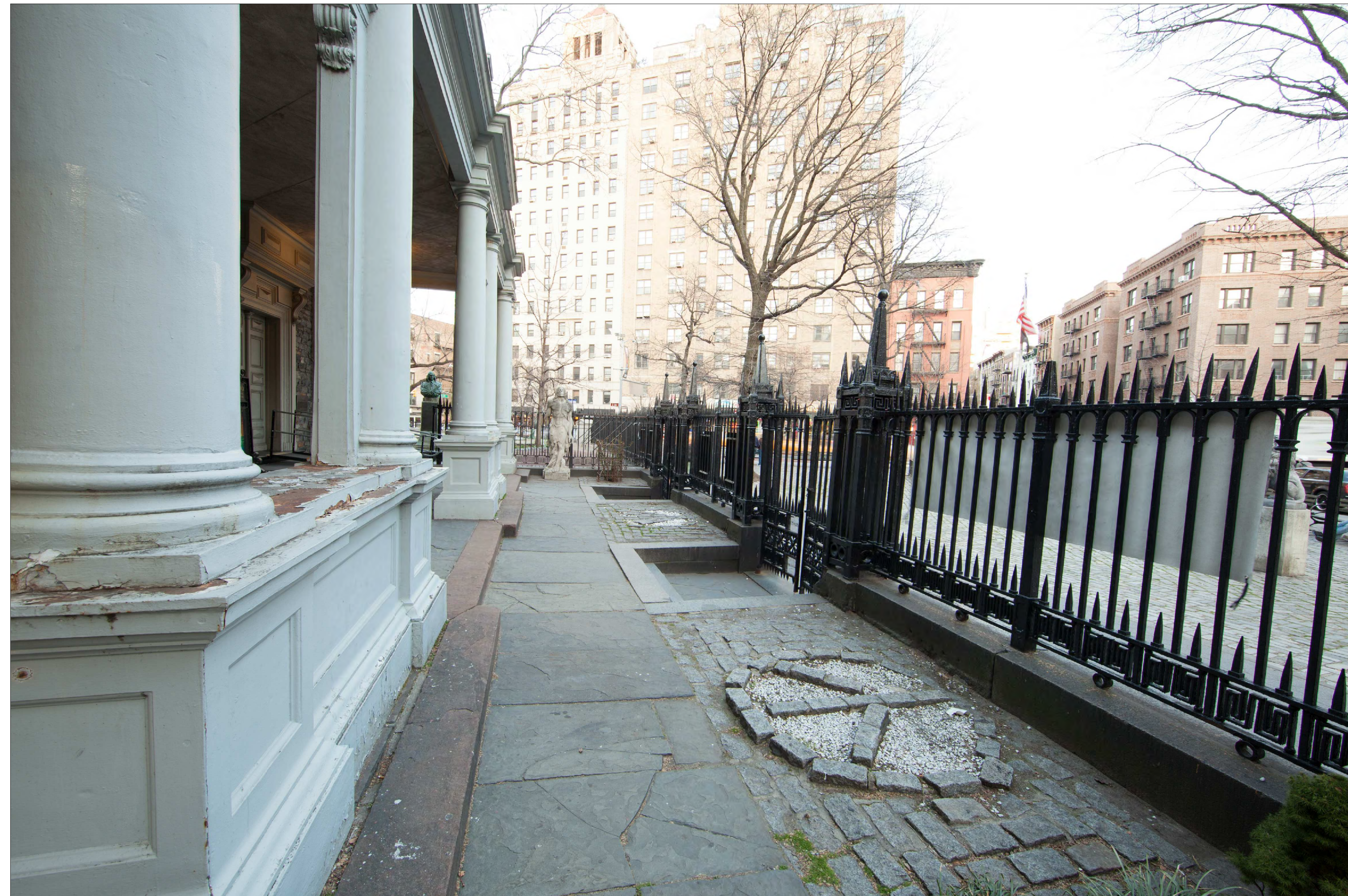
5A ENTRY RAMP - EXISTING CONDITION 2/2013 PROPOSED WORK AREA
