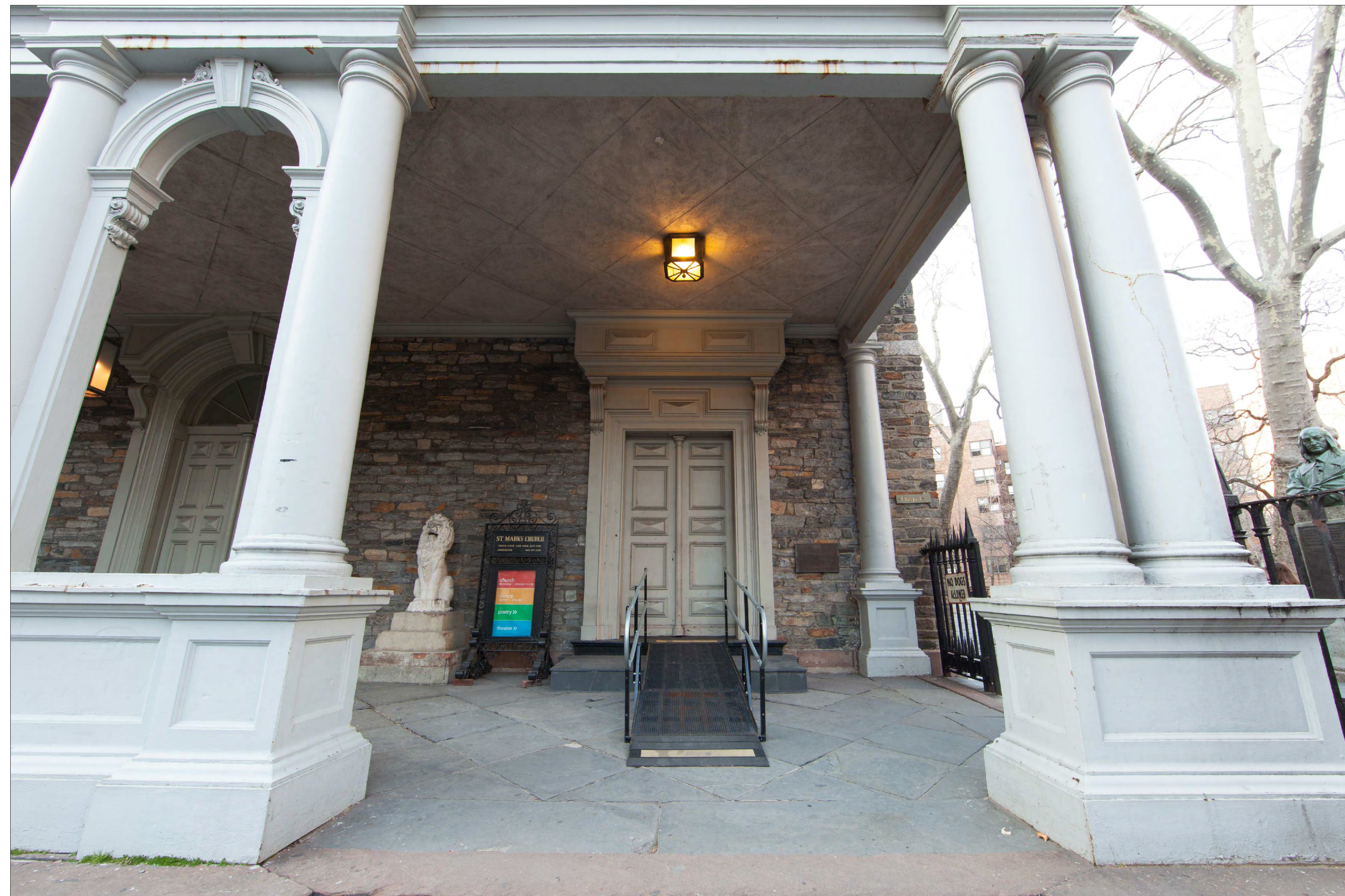
1A EAST VESTIBULE - EXISTING CONDITION 2/2013 PROPOSED WORK AREA
