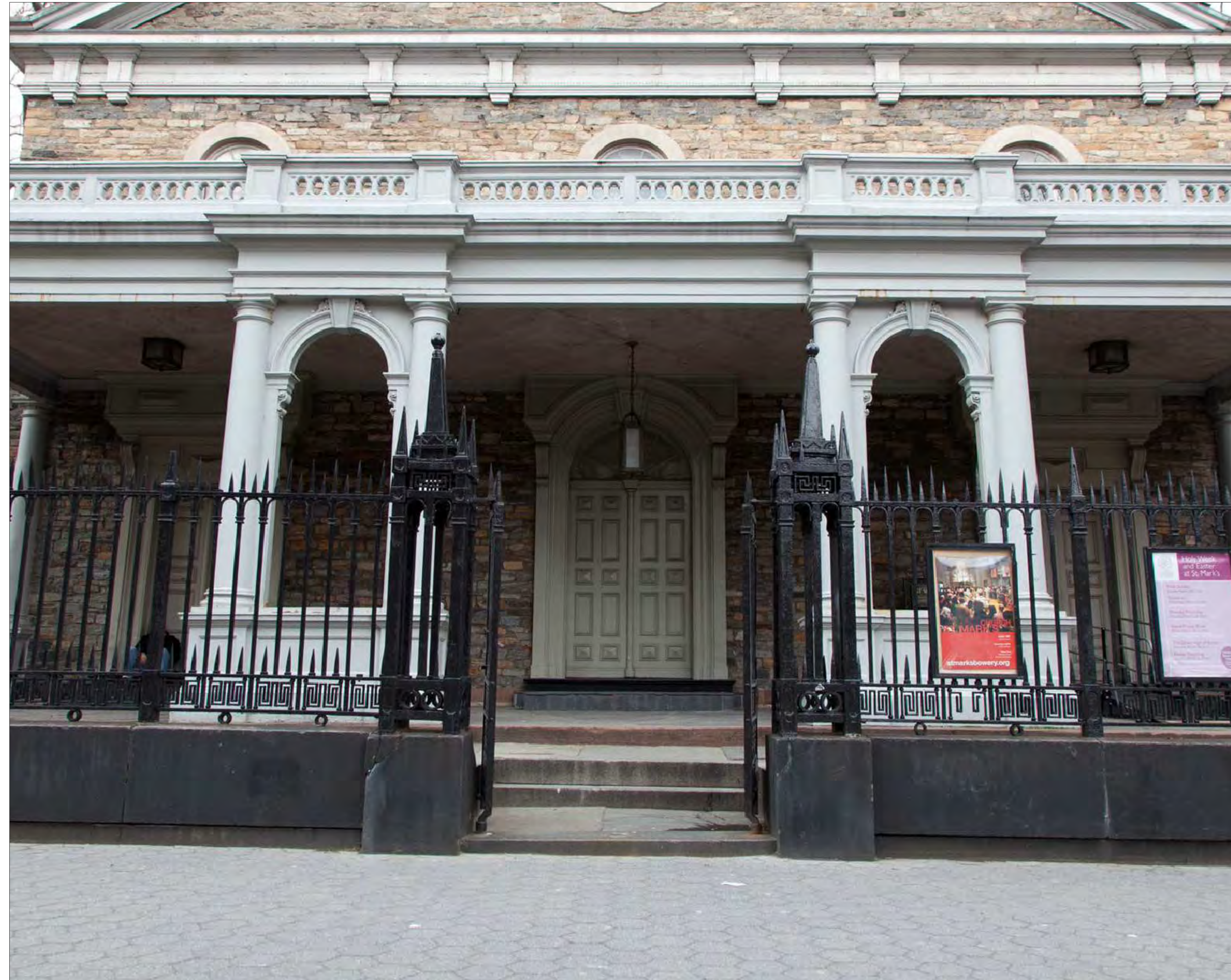
6A CENTER GATE - EXISTING CONDITION 2/2013 PROPOSED WORK AREA
