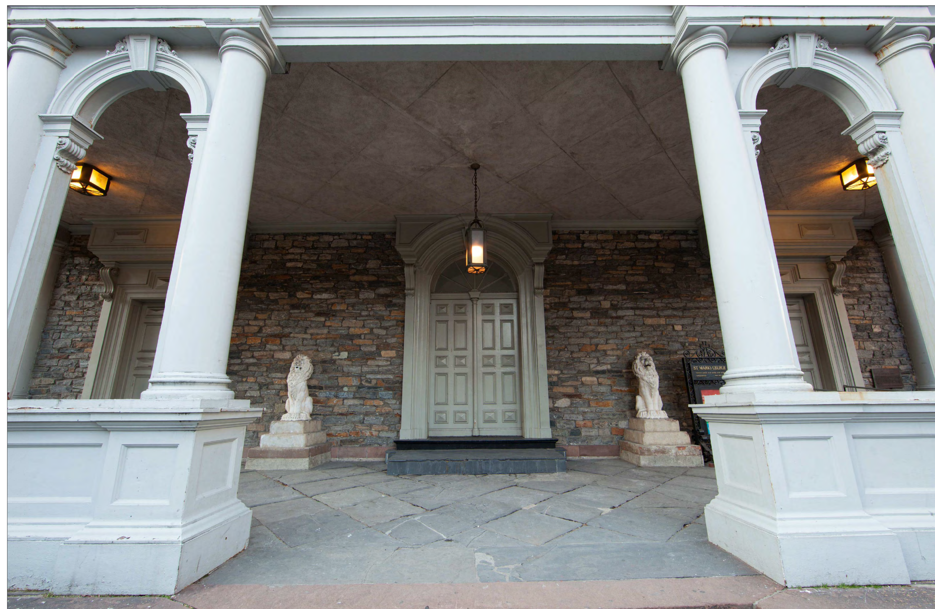
2A SANCTUARY ENTRY - EXISTING CONDITION 2/2013 PROPOSED WORK AREA
