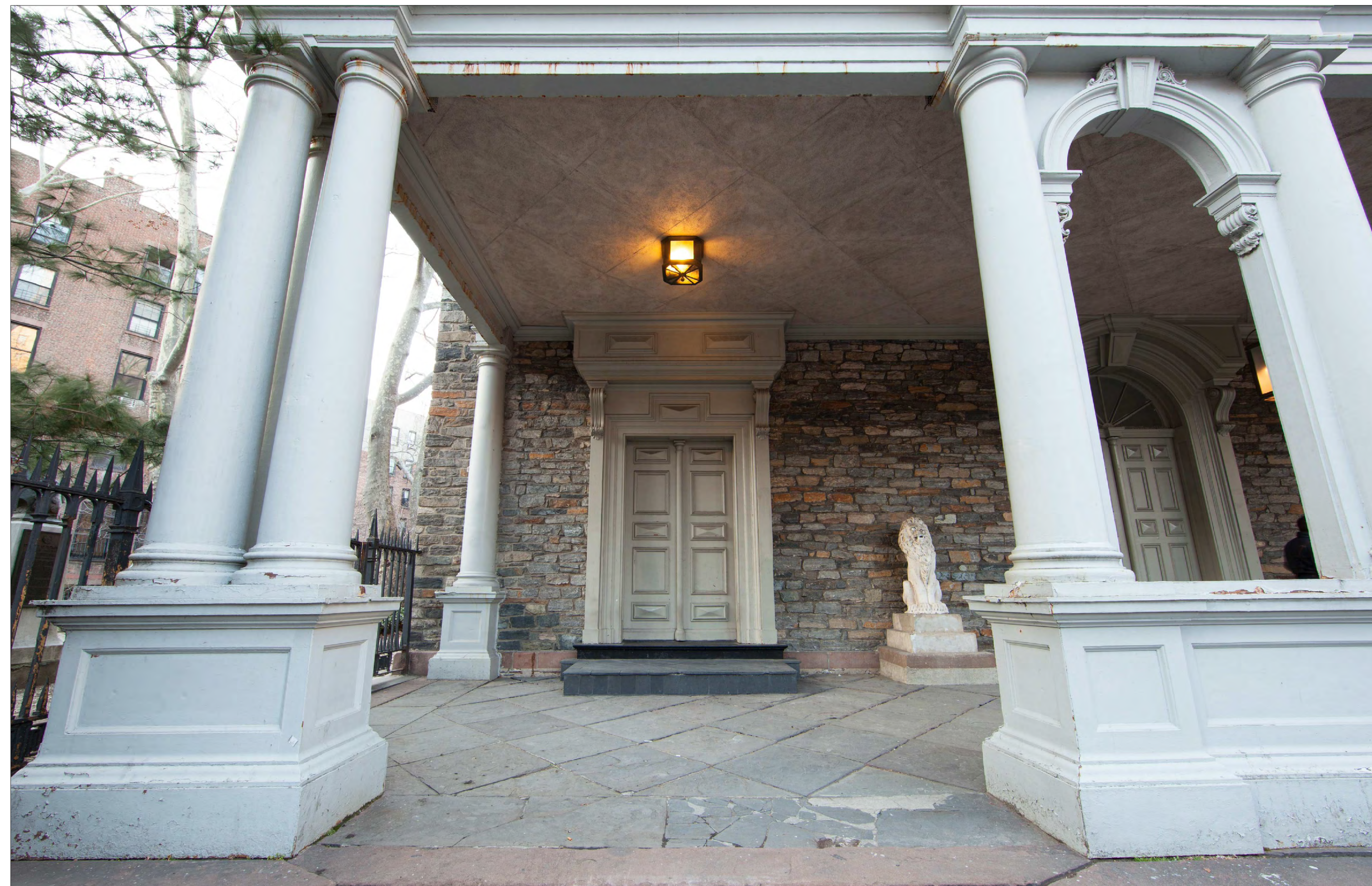
3A WEST VESTIBULE - EXISTING CONDITION 2/2013 PROPOSED WORK AREA
