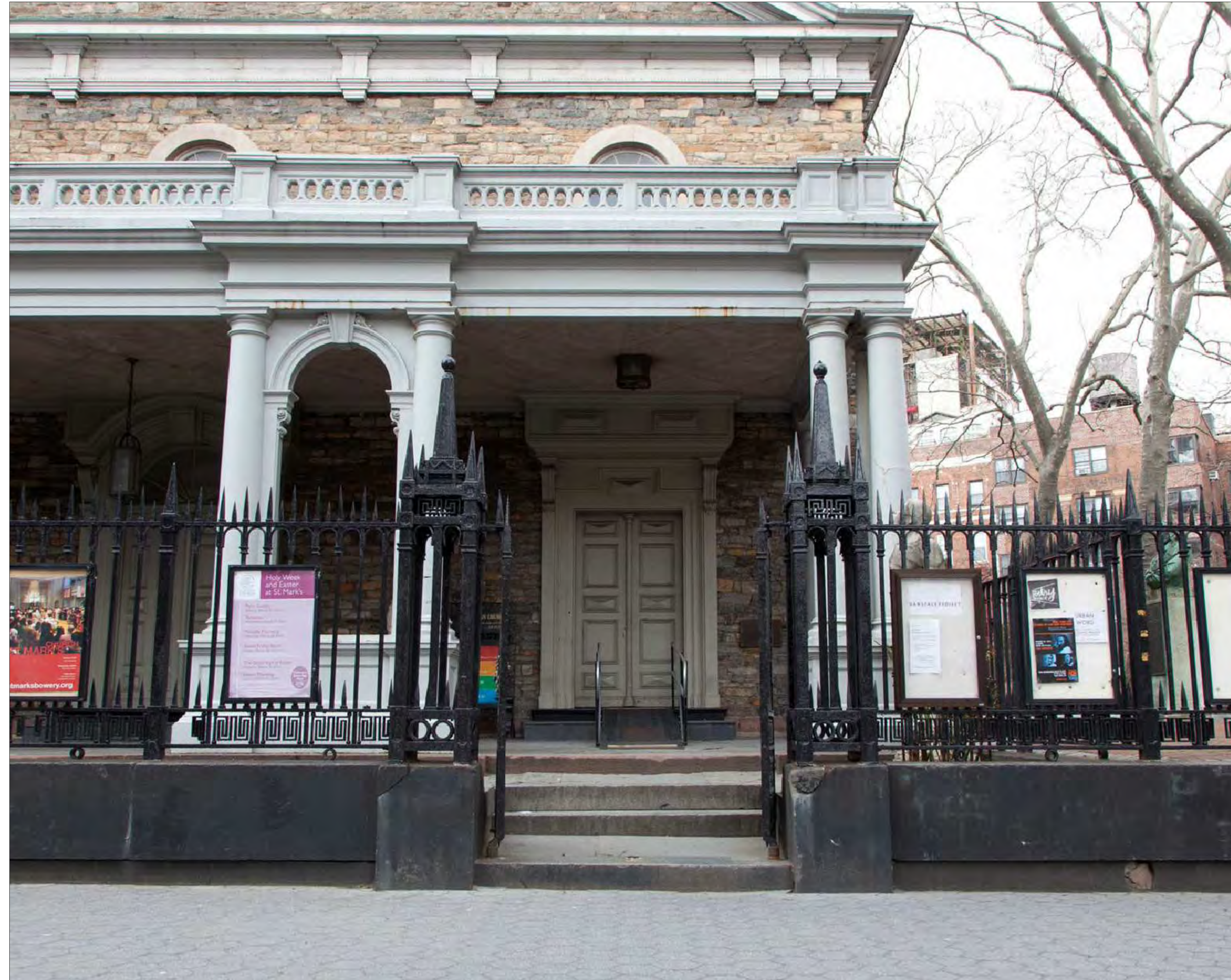
7A EAST GATE - EXISTING CONDITION 2/2013 PROPOSED WORK AREA
