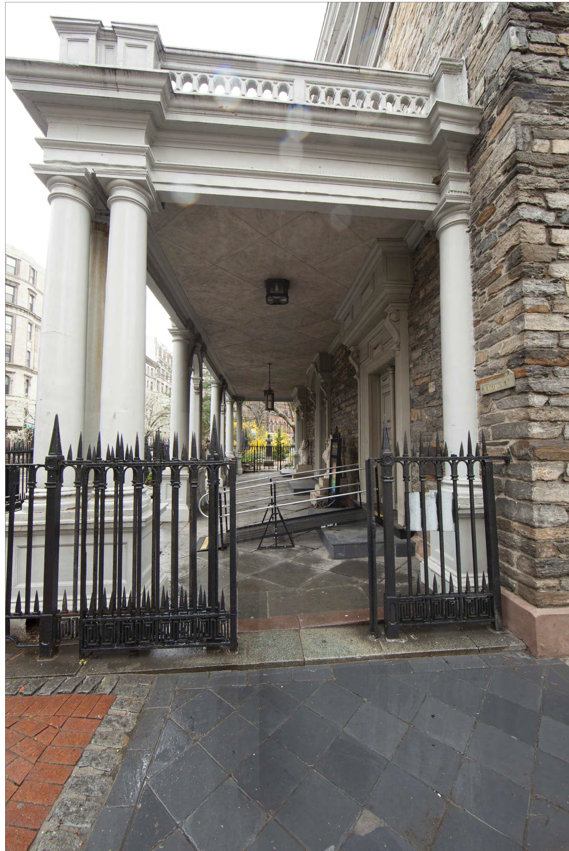
4A EAST ELEVATION - EXISTING CONDITION 2/2013 PROPOSED WORK AREA
