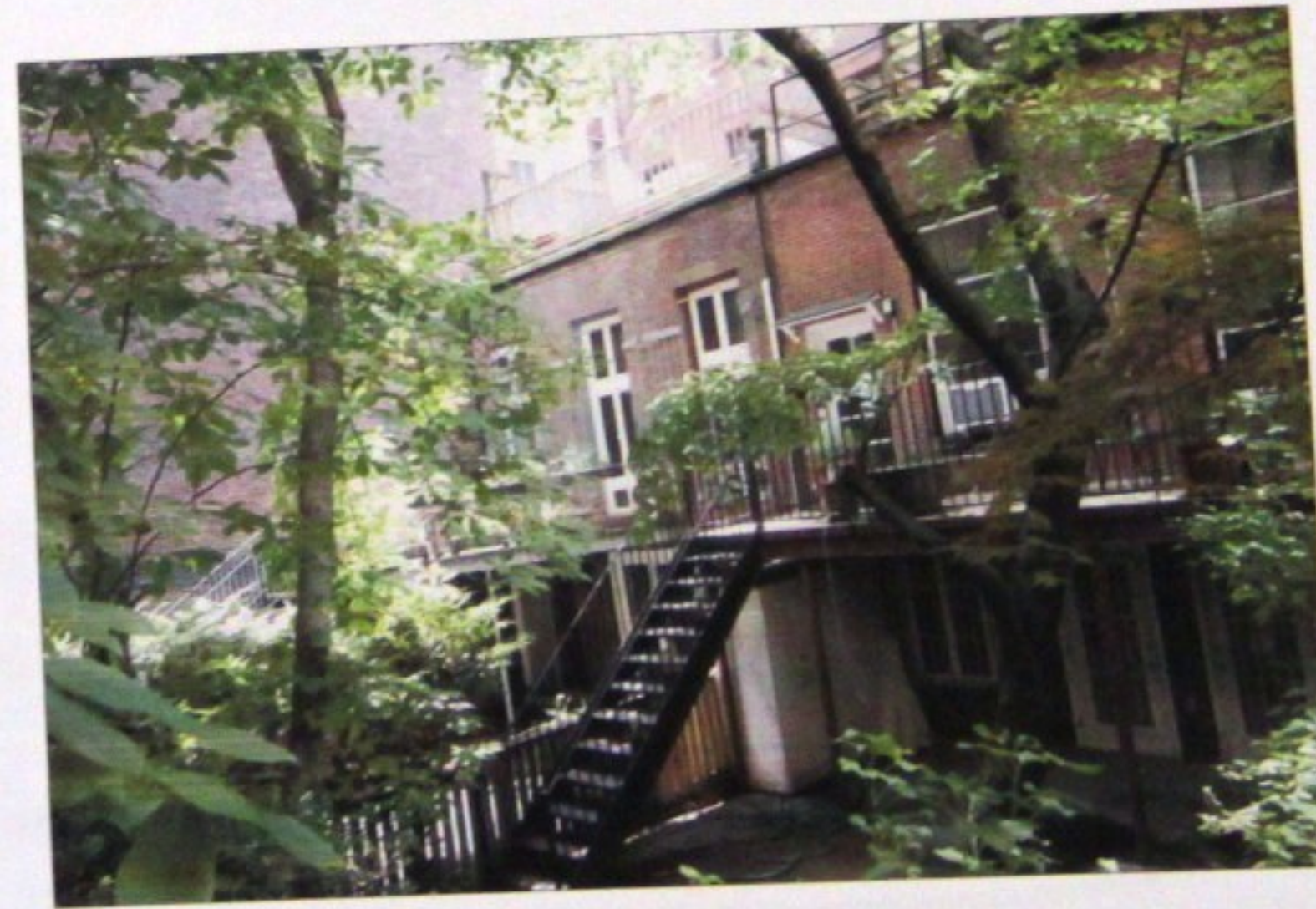
03 REAR ELEVATION @ 129 & 127 W.12th ST, EXISTING L-006 N/A
