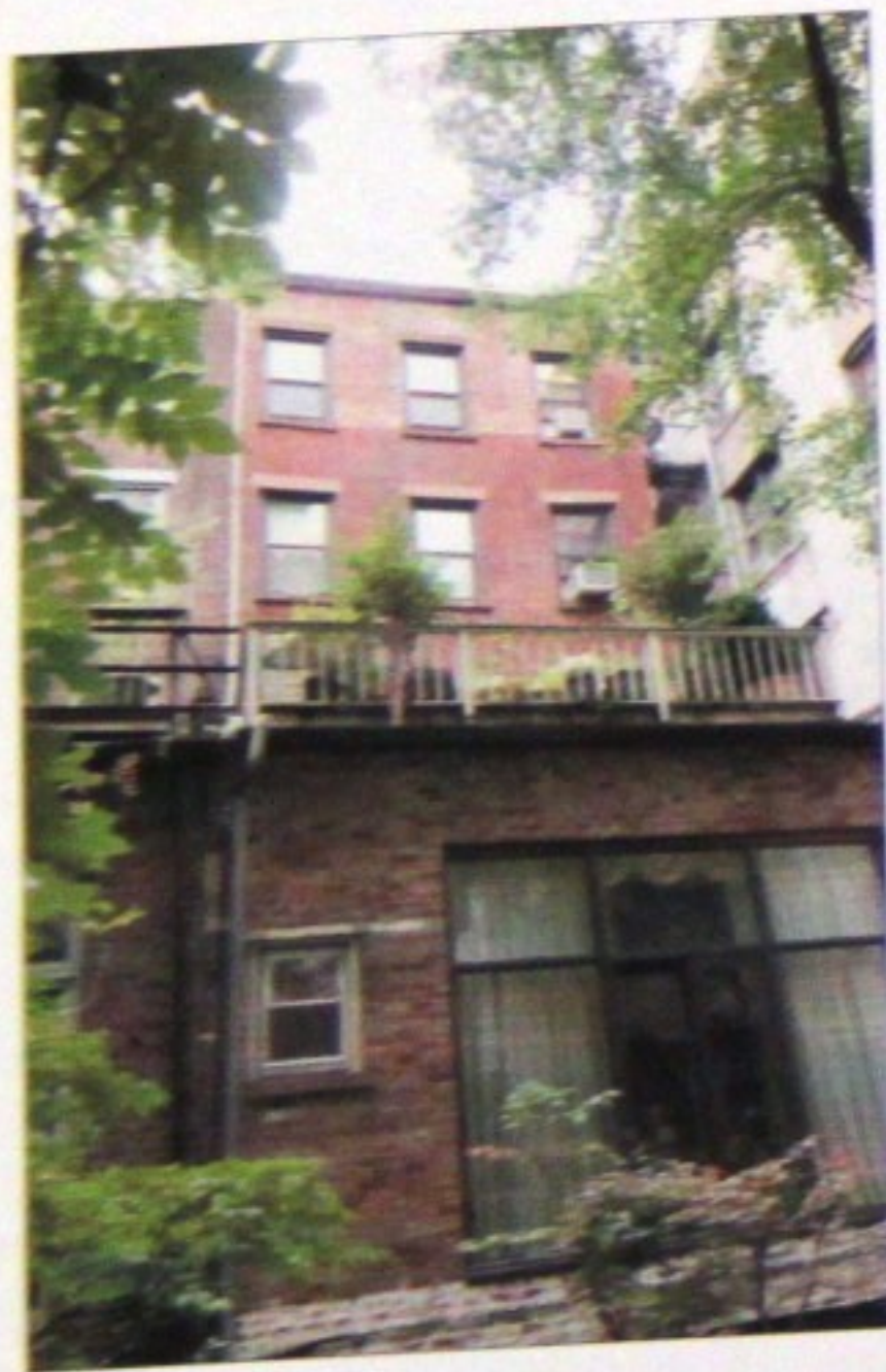
01 REAR ELEVATION @ 135 W.12th ST, EXISTING L-006 N/A
