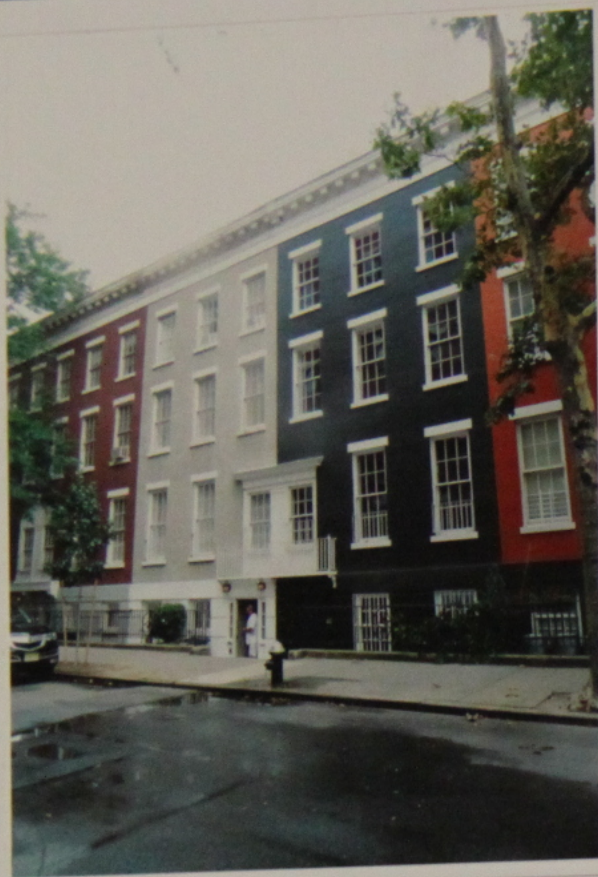
1 90 MACDOUGAL STREET - EXISTING PAINTED FRONT FACADE
