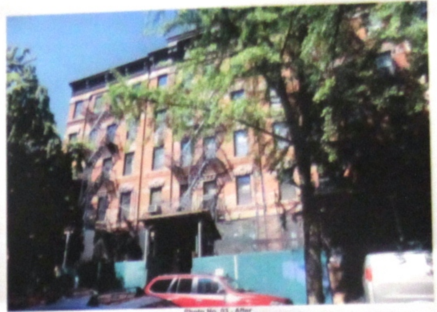
Photo No. 03 - After
