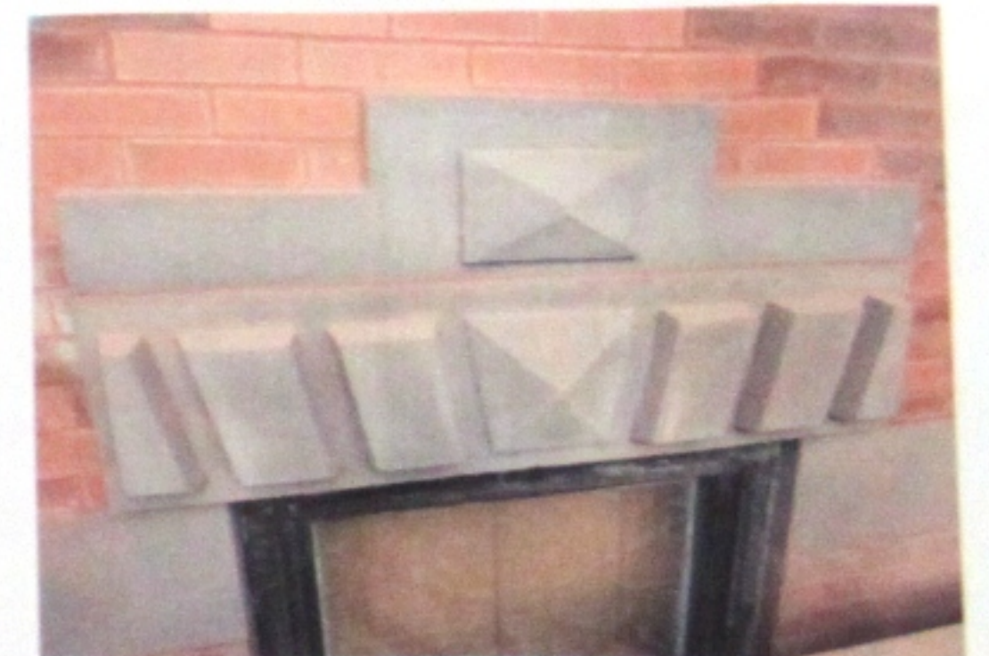
Photo No. 07 - After
