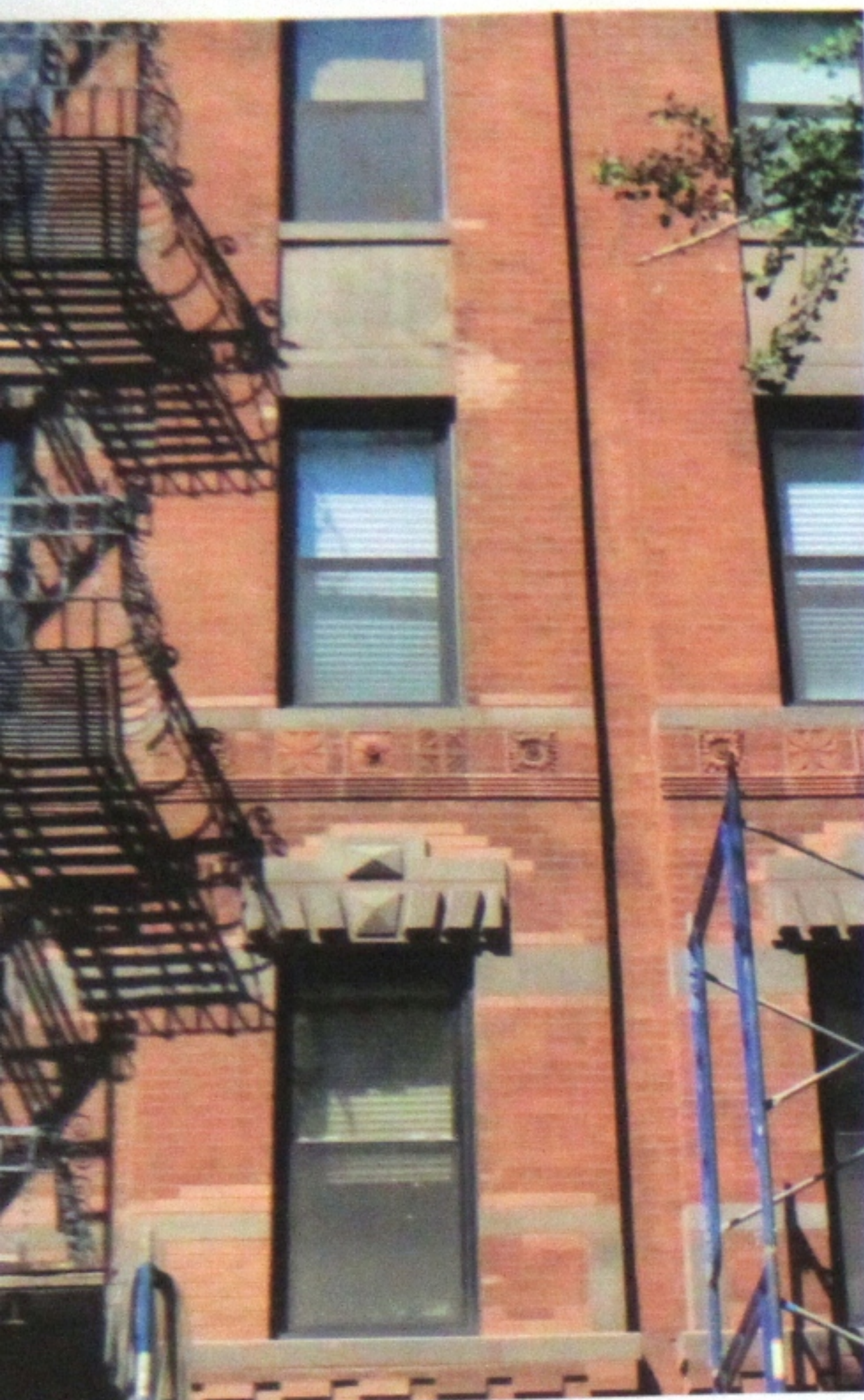
Photo No. 05 - After
