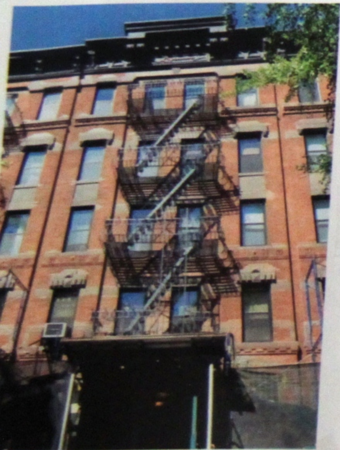
Photo No. 04 - After
