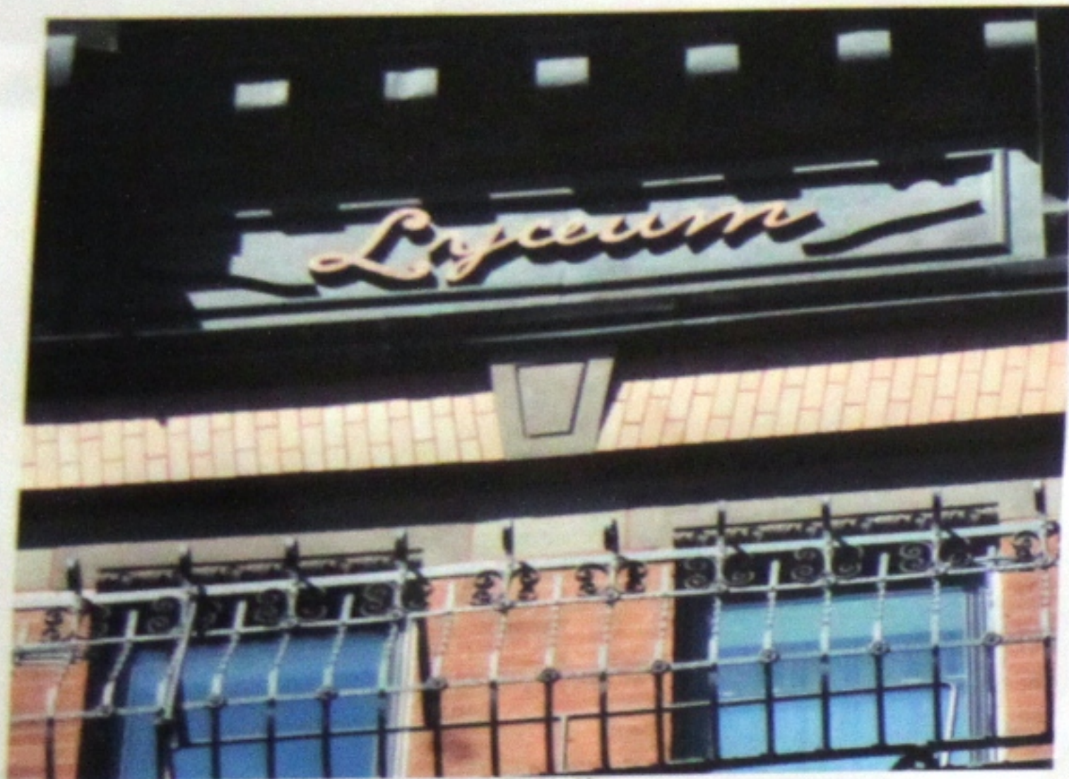
Photo No. 01 - After
