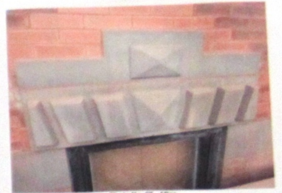
Photo No. 07 - After
