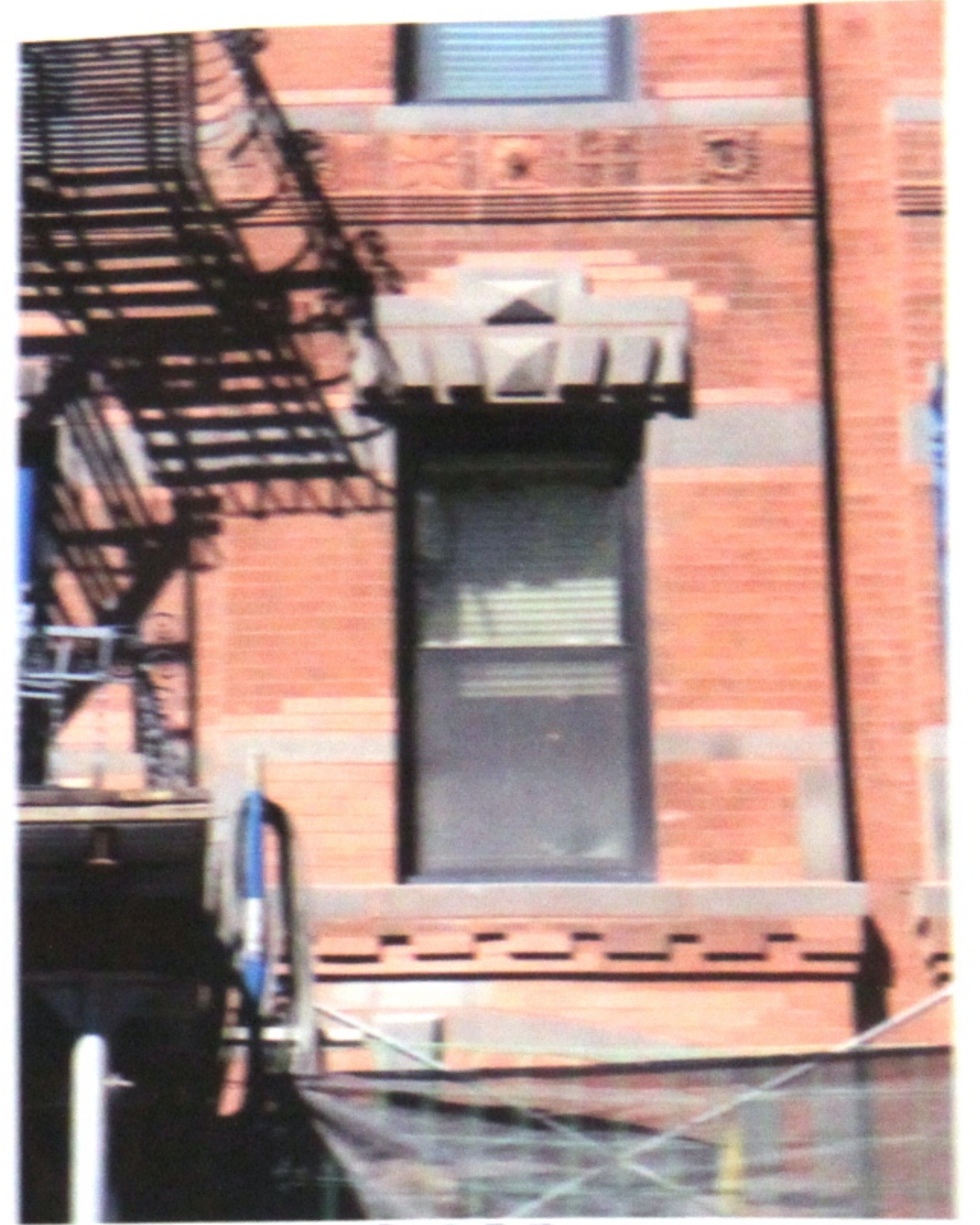
Photo No. 26 - after
