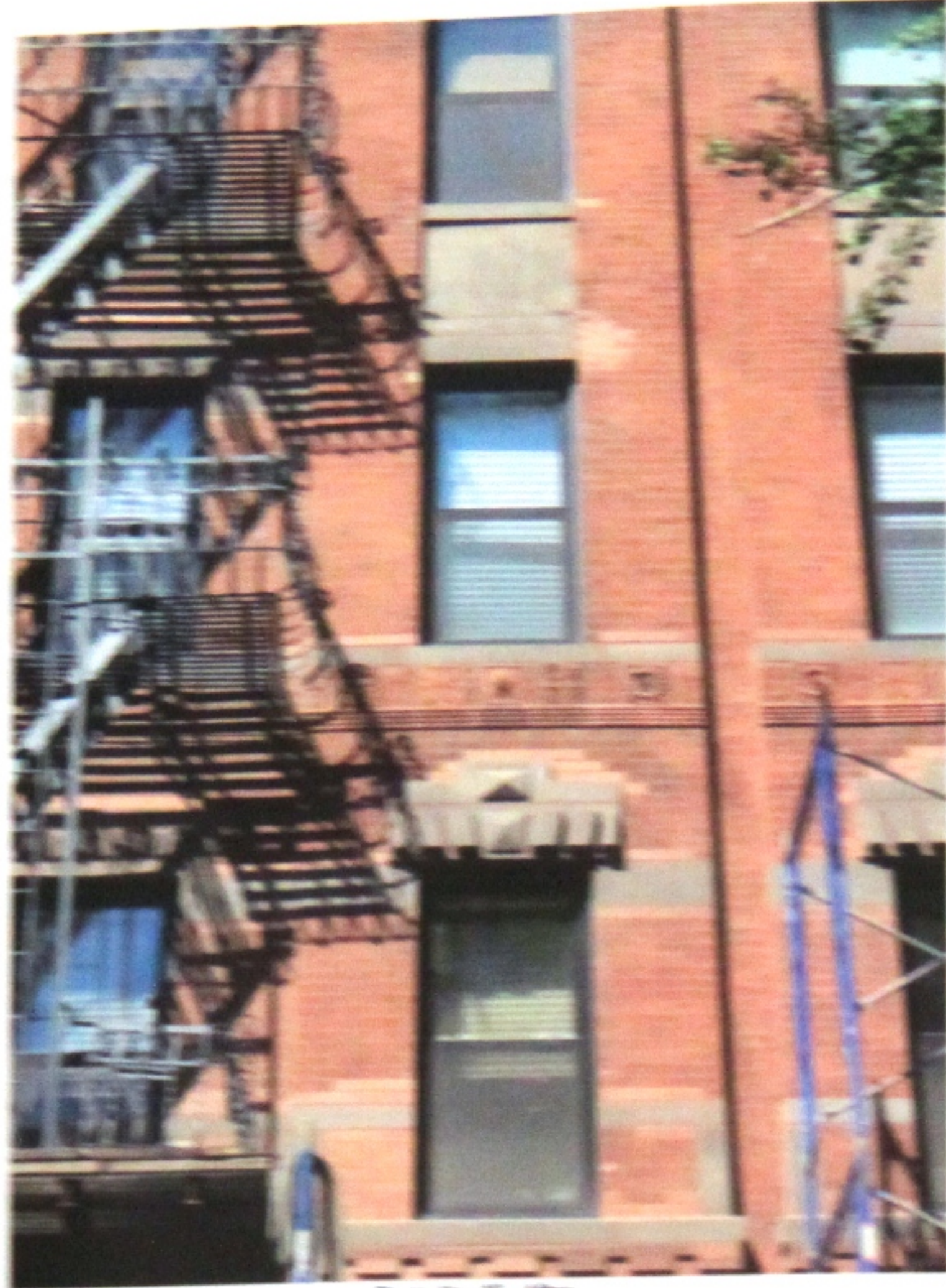
Photo No. 25 - after
