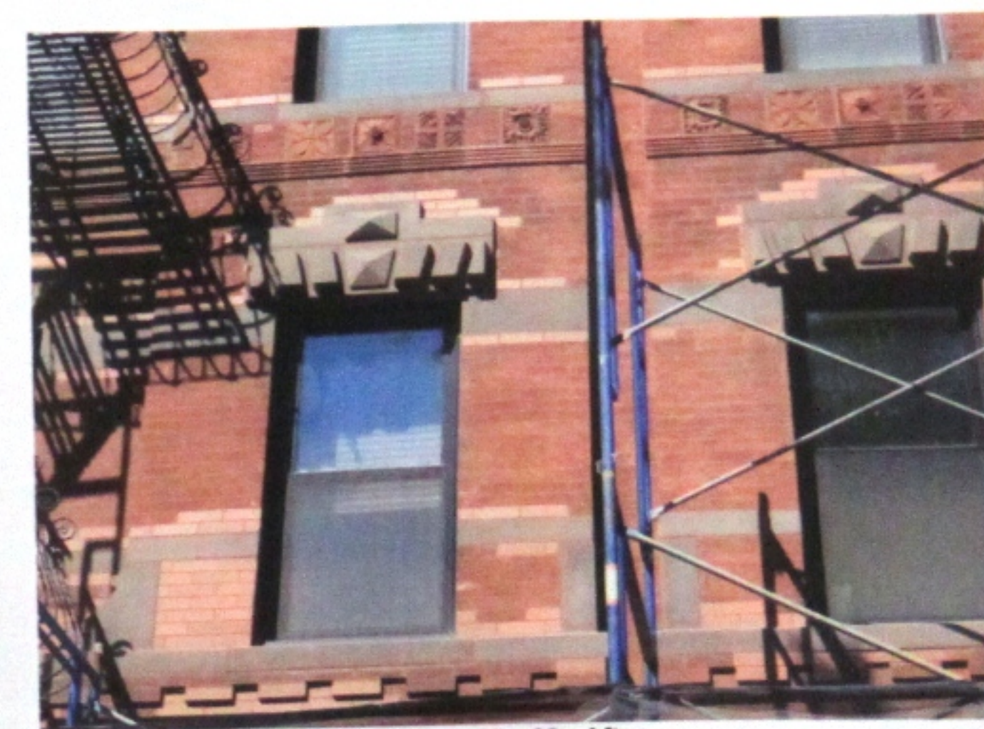
Photo No. 08 - After
