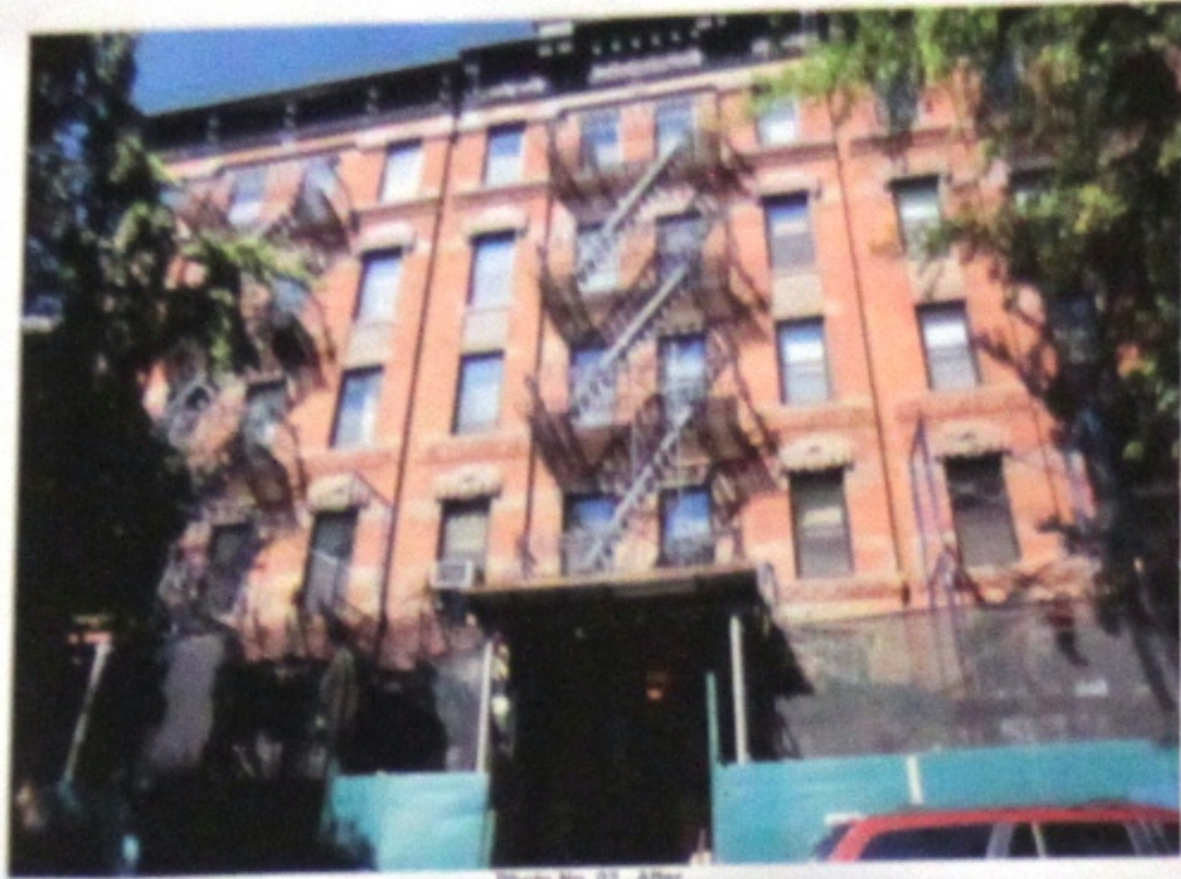
Photo No. 02 - After
