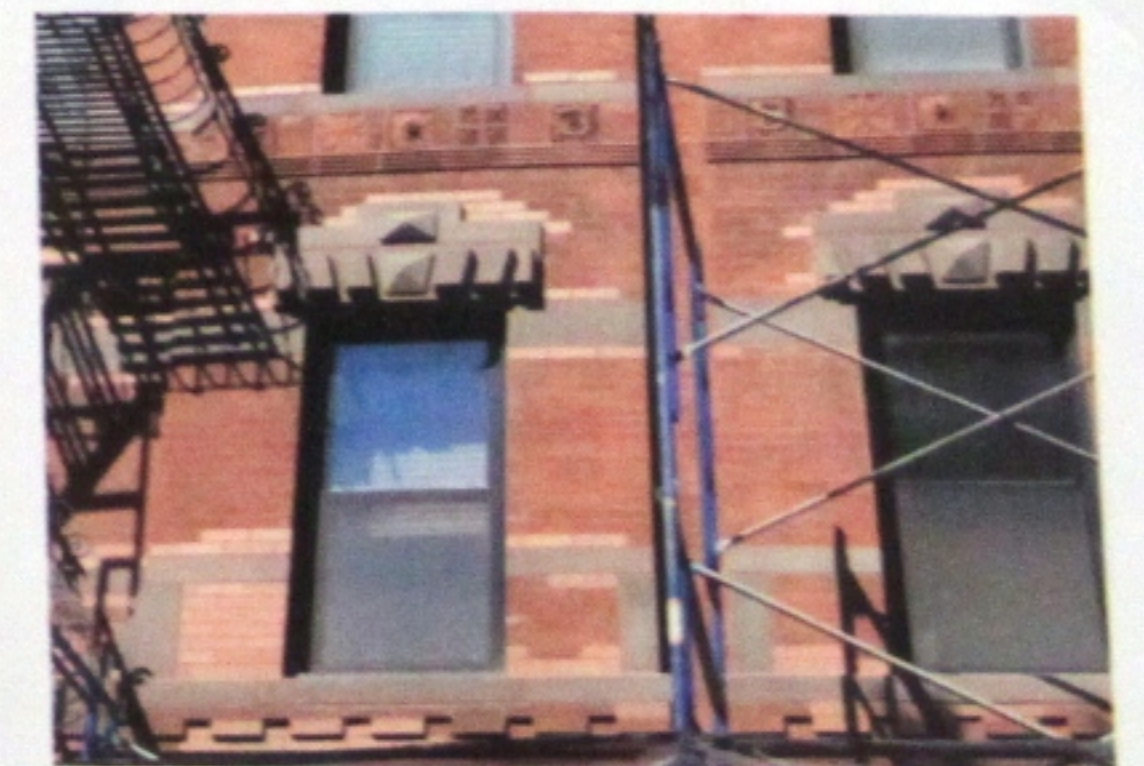
Photo No. 08 - After
