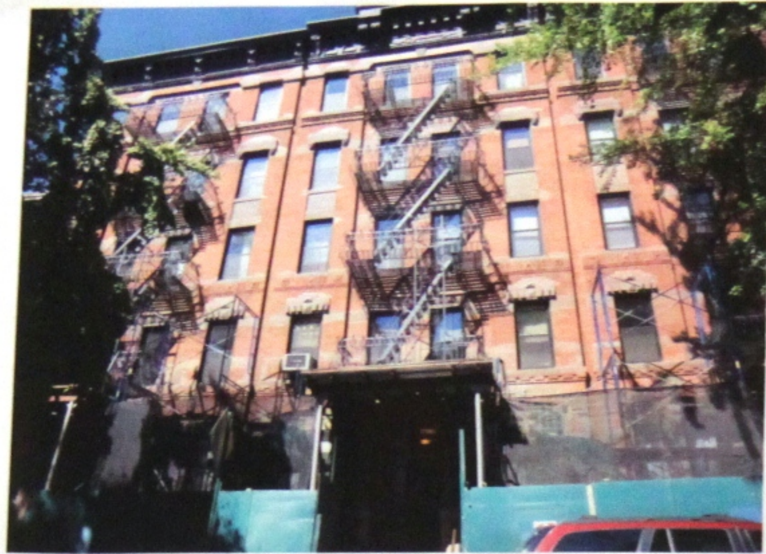
Photo No. 02 - After
