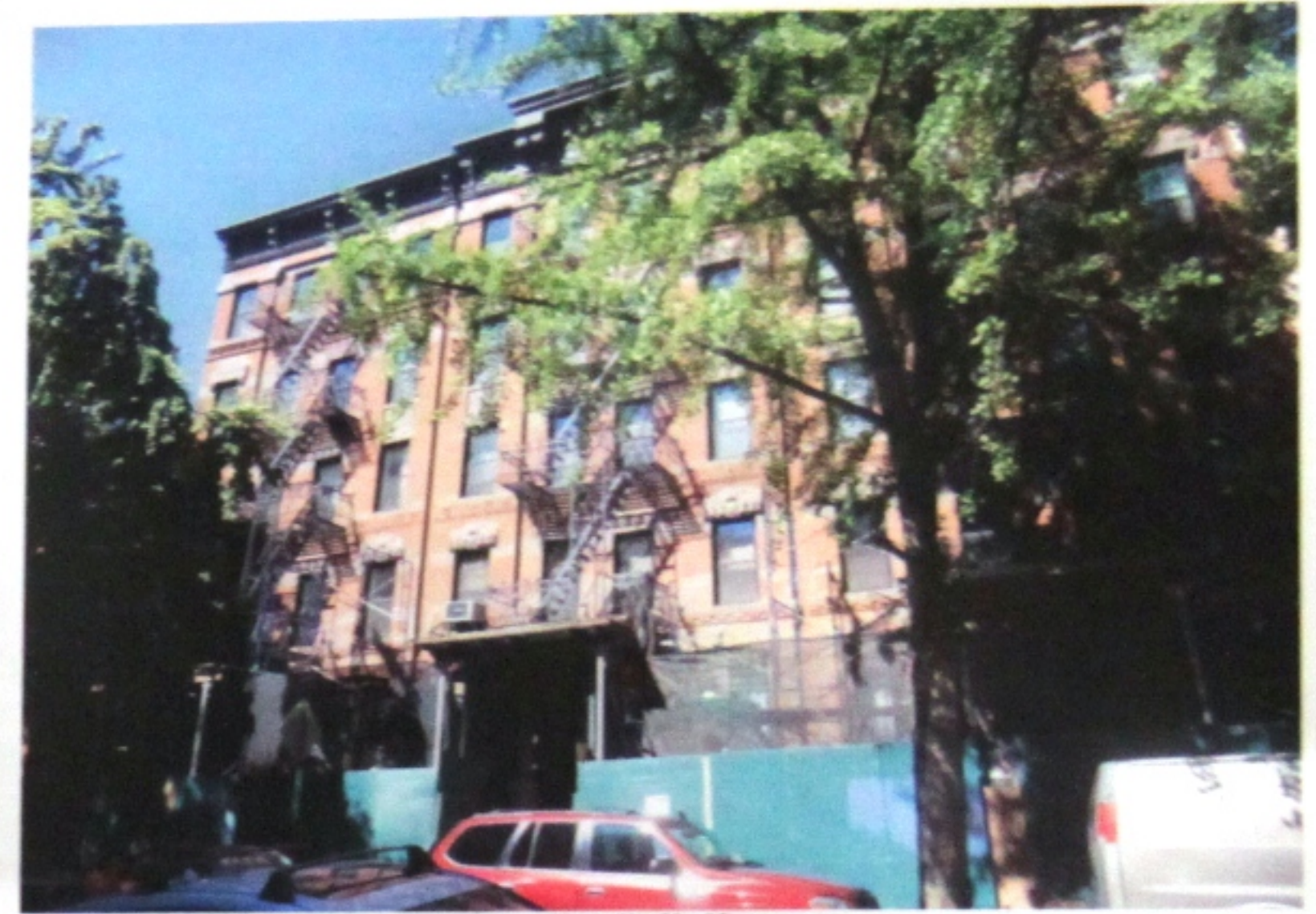
Photo No. 03 - After
