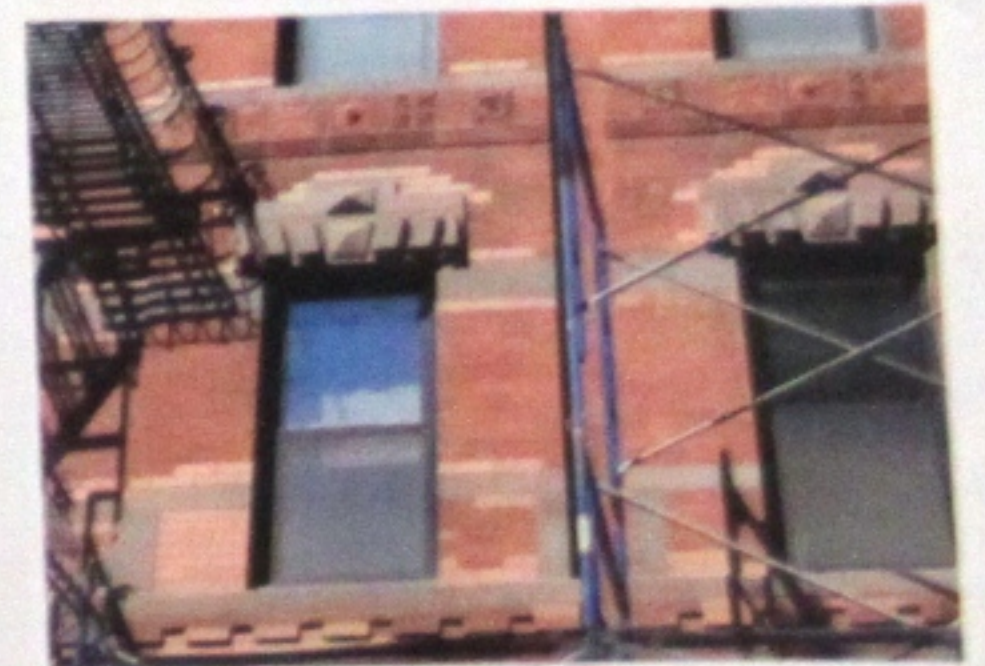
Photo No. 08 - After
