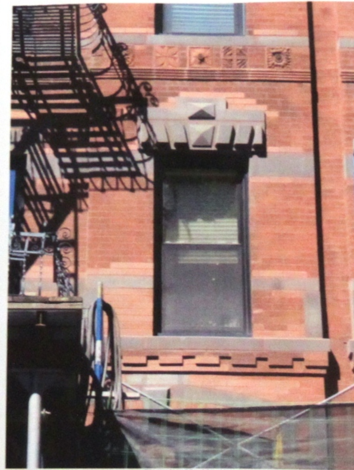
Photo No. 06 - After
