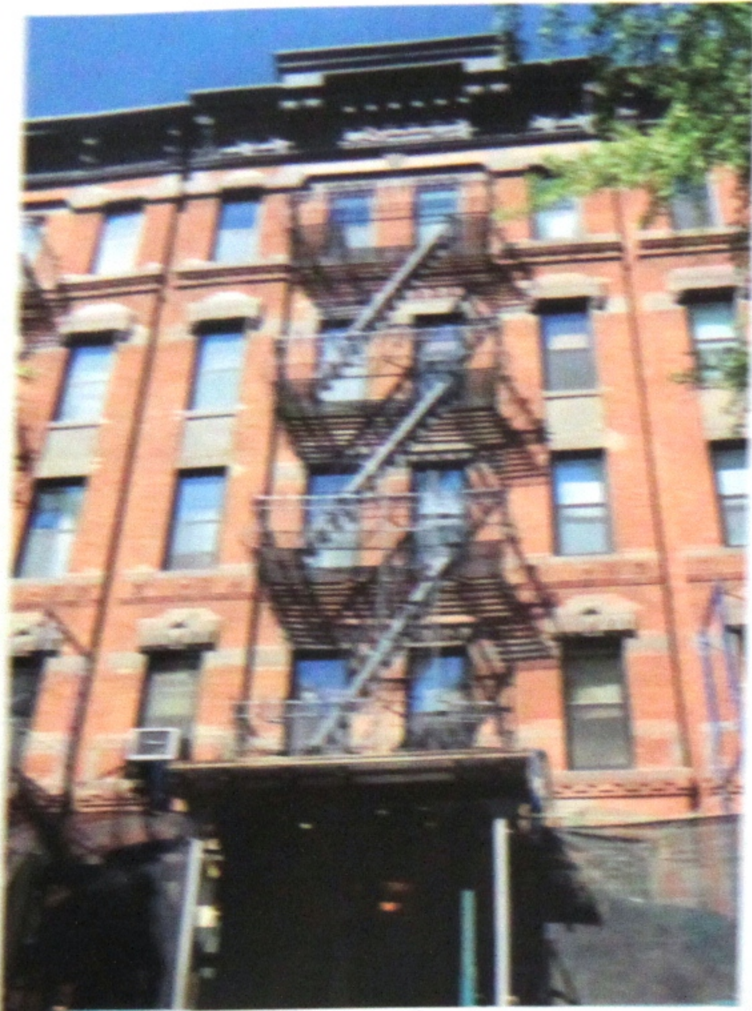
Photo No. 24 - after
