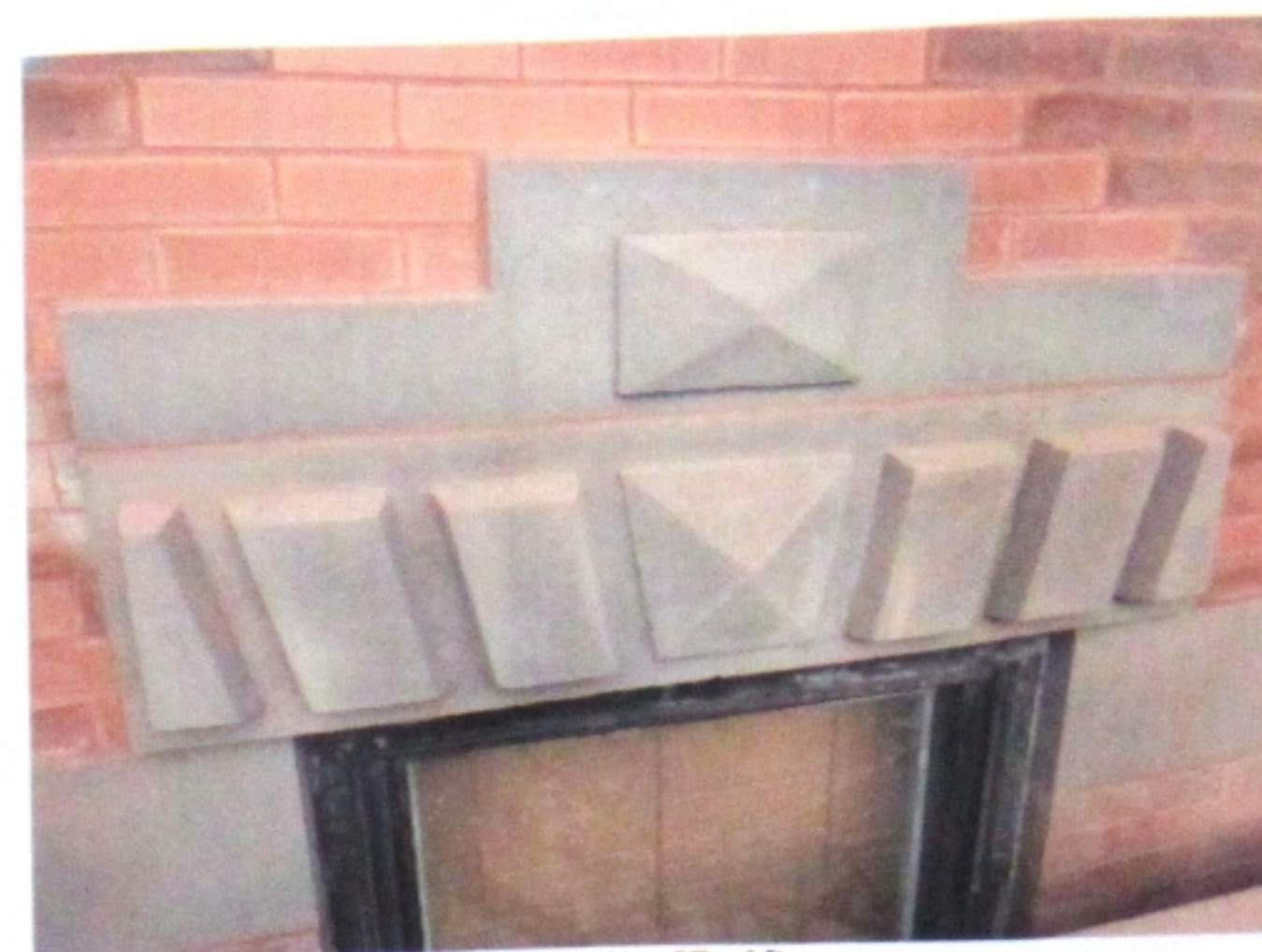
Photo No. 07 - After
