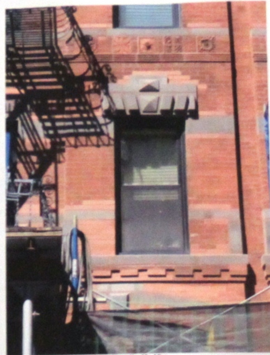
Photo No. 06 - After
