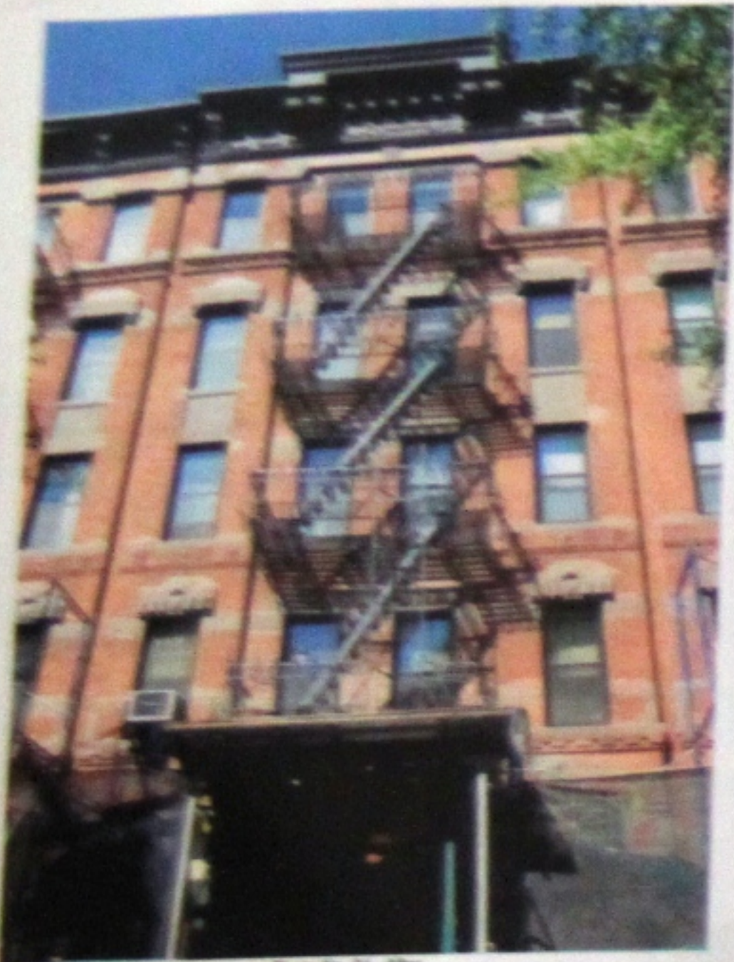
Photo No. 04 - After
