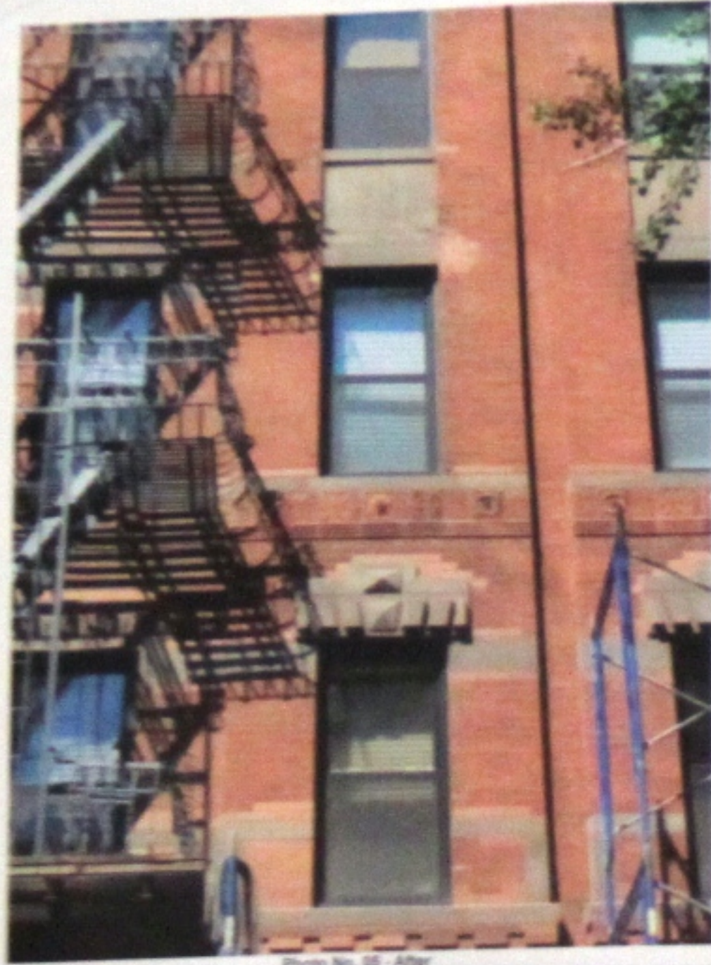
Photo No. 05 - After
