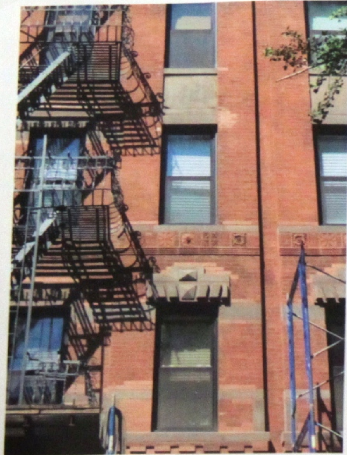
Photo No. 05 - After
