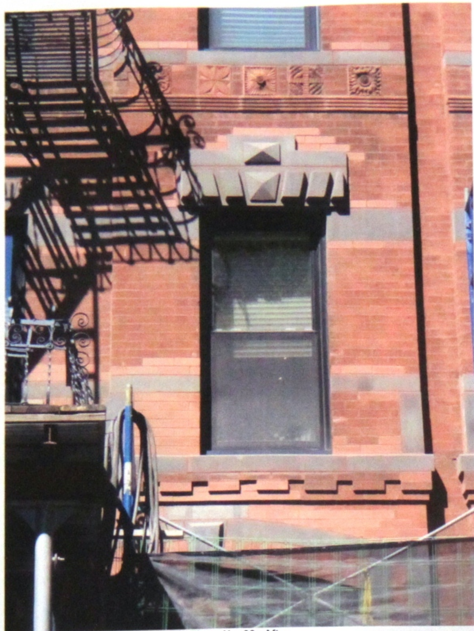
Photo No. 06 - After
