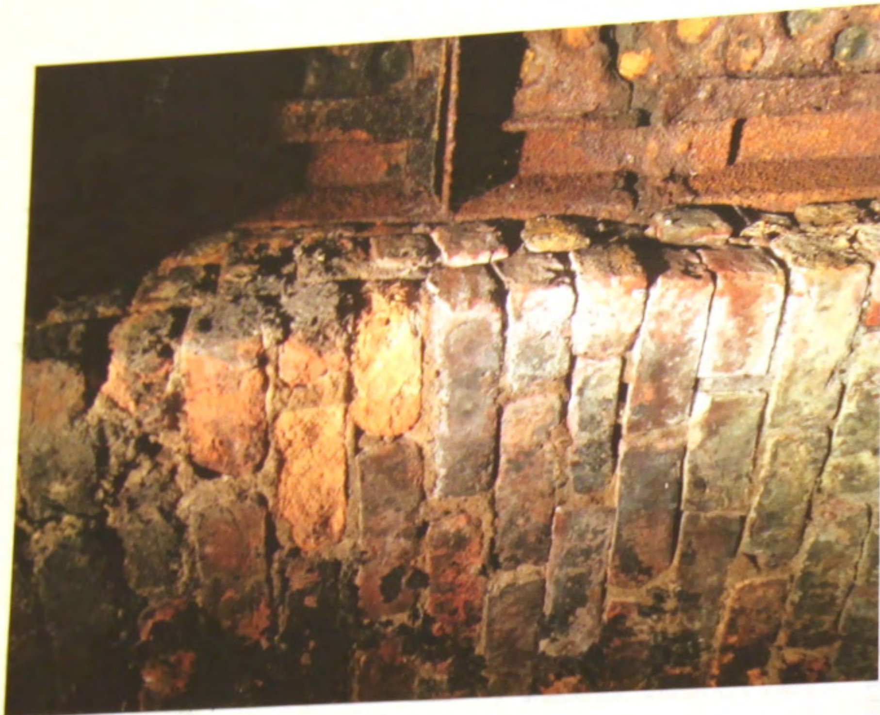
PHOTO 1 UNDERSIDE OF VAULT AT EDGE OF BRICK ARCH
