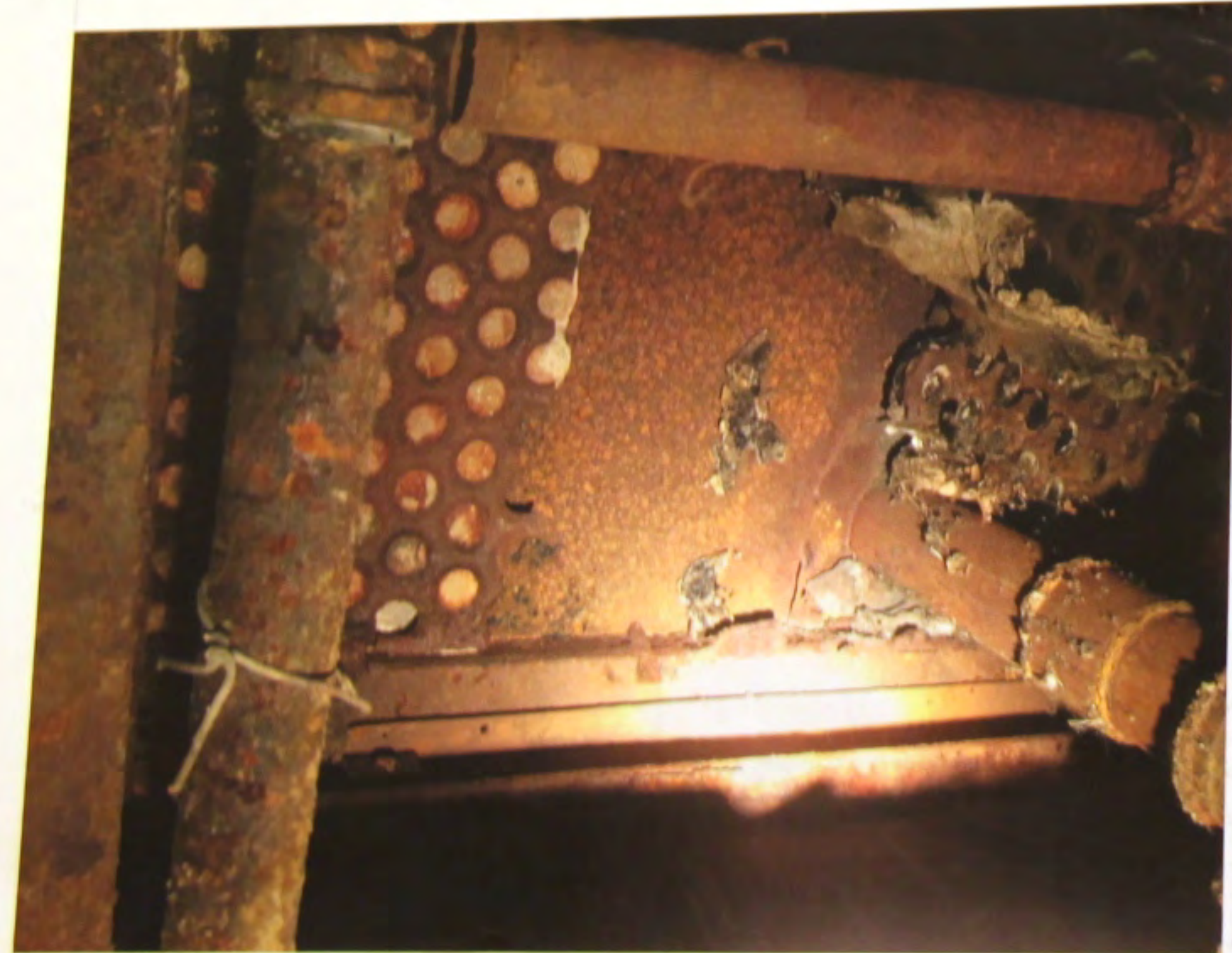
PHOTO 3 UNDERSIDE OF VAULT AT STANDPIPE PENETRATION
