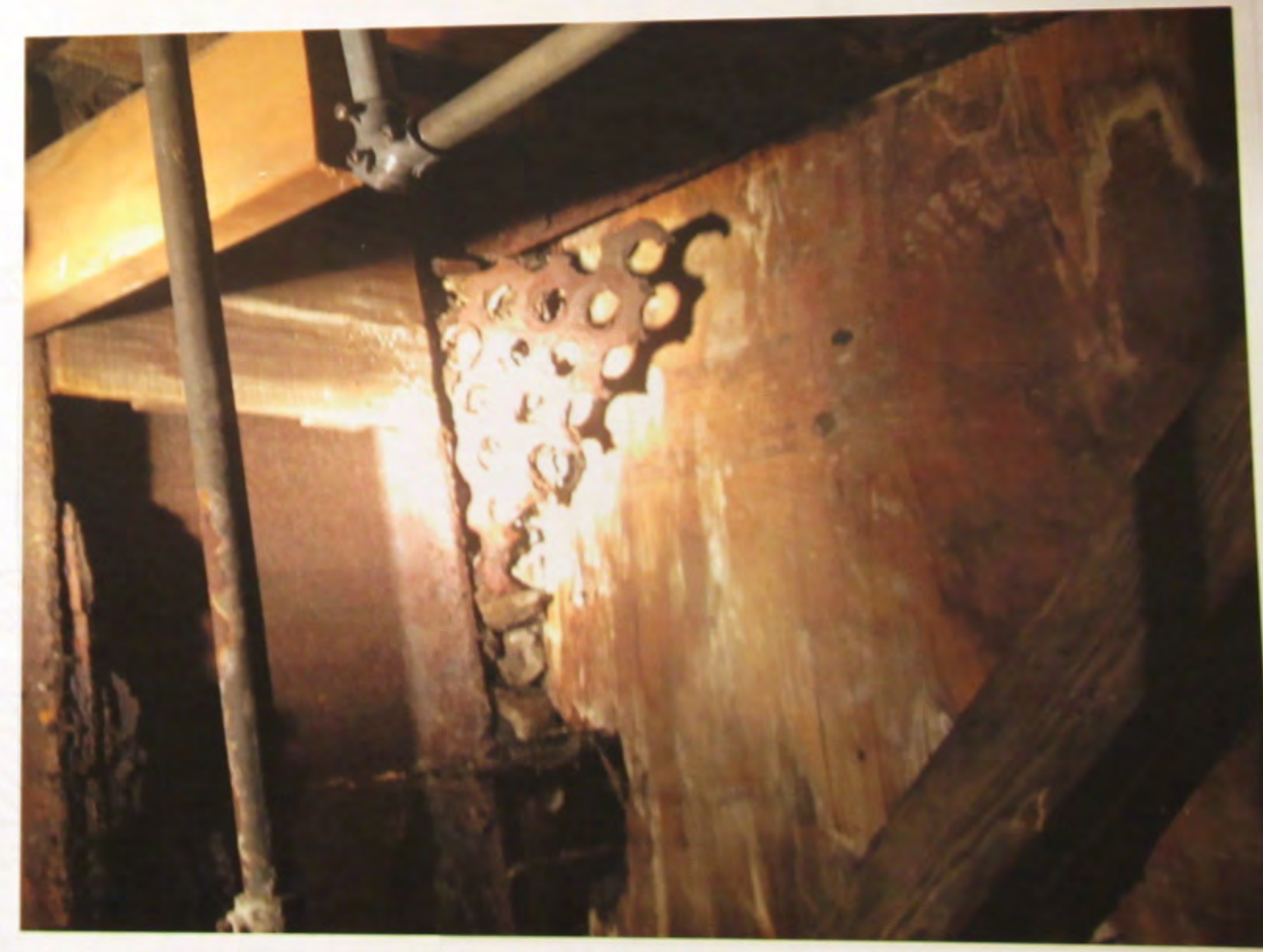
PHOTO 4 UNDERSIDE OF VAULT AT CONCRETE RAMP
