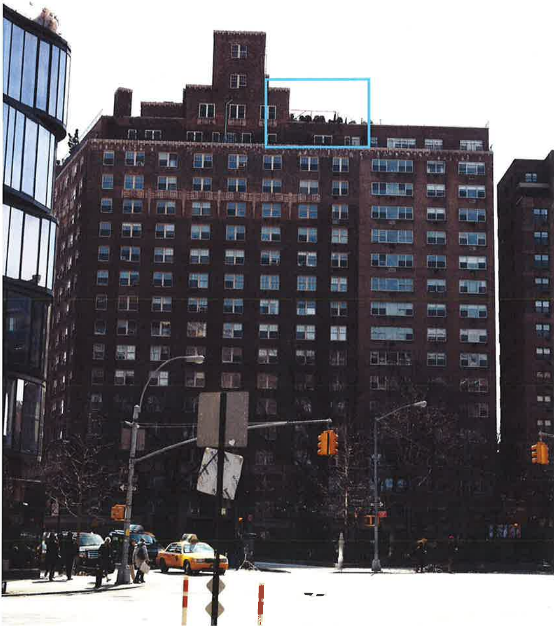
B: 14 STREET AND 8TH AVE (VISIBLE)
