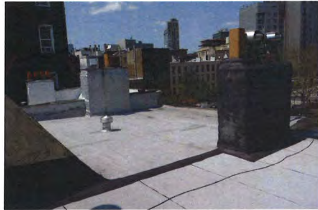
CURRENT ROOFTOP VIEW - NORTH - 44 HORATIO STREET
