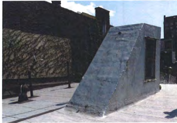
CURRENT ROOFTOP VIEW - SOUTH - 46 HORATIO STREET
