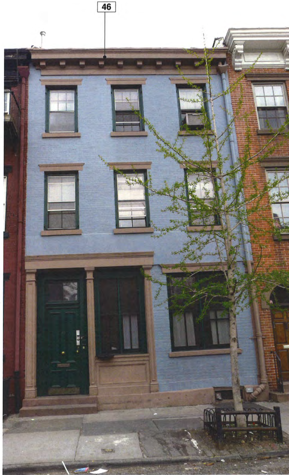
CURRENT CONDITIONS -2015 PHOTO OF 46 HORATIO STREET
