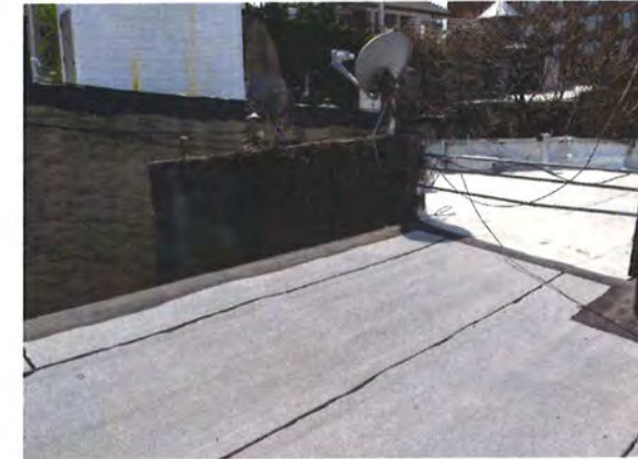
CURRENT ROOFTOP VIEW - WEST - 44 HORATIO STREET
