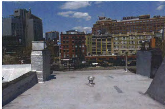
CURRENT ROOFTOP VIEW - NORTH - 46 HORATIO STREET
