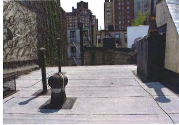
CURRENT ROOFTOP VIEW - SOUTH - 44 HORATIO STREET
