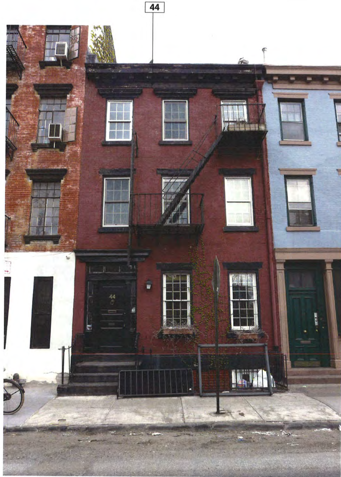
CURRENT CONDITIONS -2015 PHOTO OF 44 HORATIO STREET
