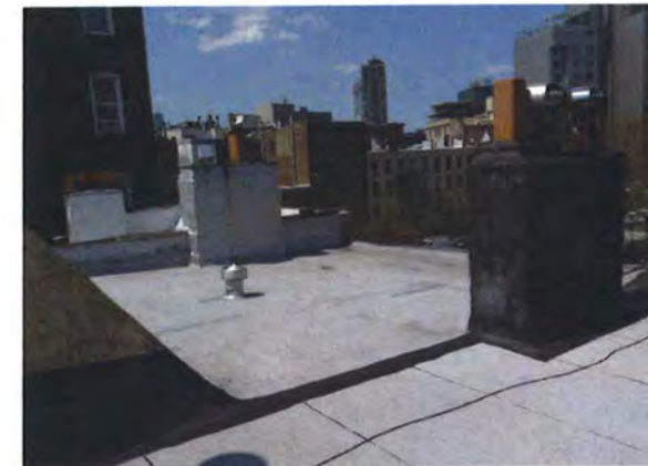
CURRENT ROOFTOP VIEW - NORTH EAST - 46 HORATIO STREET
