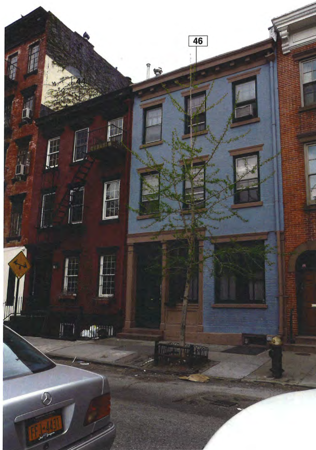
EXISTING CONDITION - 44&46 HORATIO STREET
