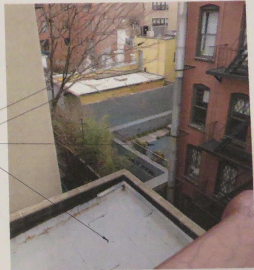
5 REAR YARD PHOTO - BLOCK REAR ADDITIONS NTS
