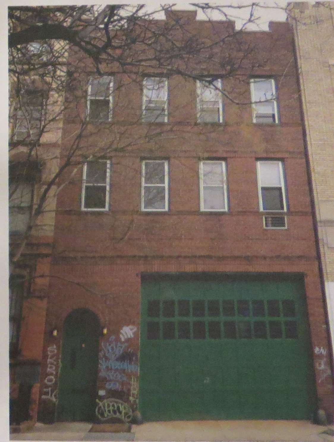
4 EXISTING FRONT FACADE PHOTO - 2013 NTS
