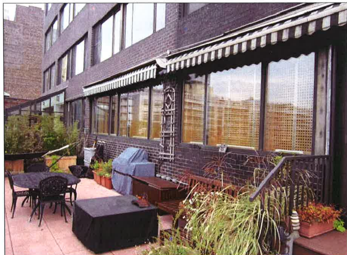
EXISTING CONDITION, TERRACE
