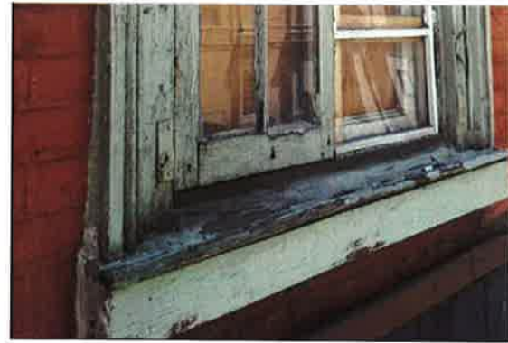
8 EXISTING WINDOW SILL + ENFRAMENT PHOTO NTS
