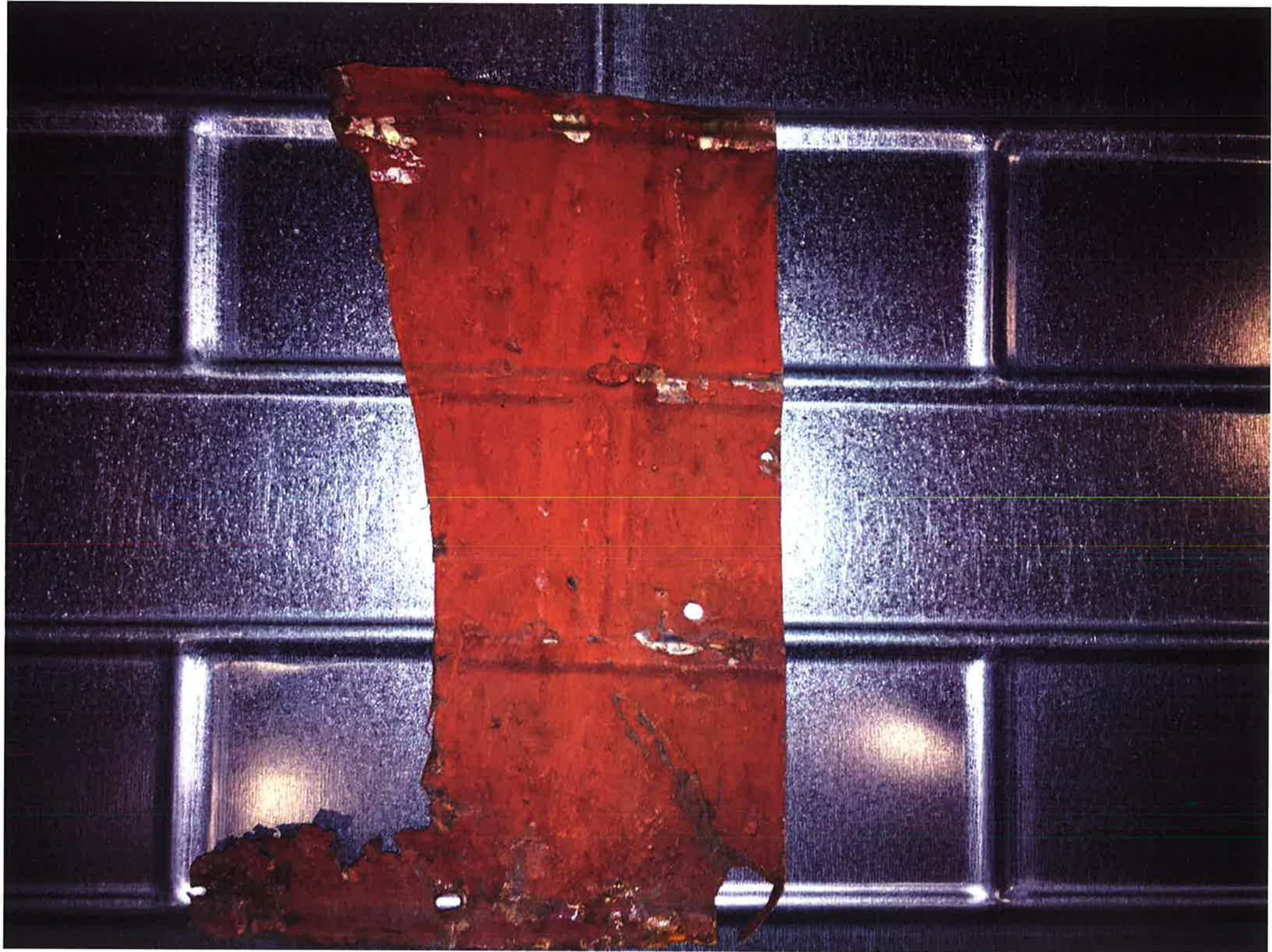
ORIGINAL PAINTED PRESSED METAL OVER PROPOSED PRESSED METAL BY W.F. NORMAN CORP.
