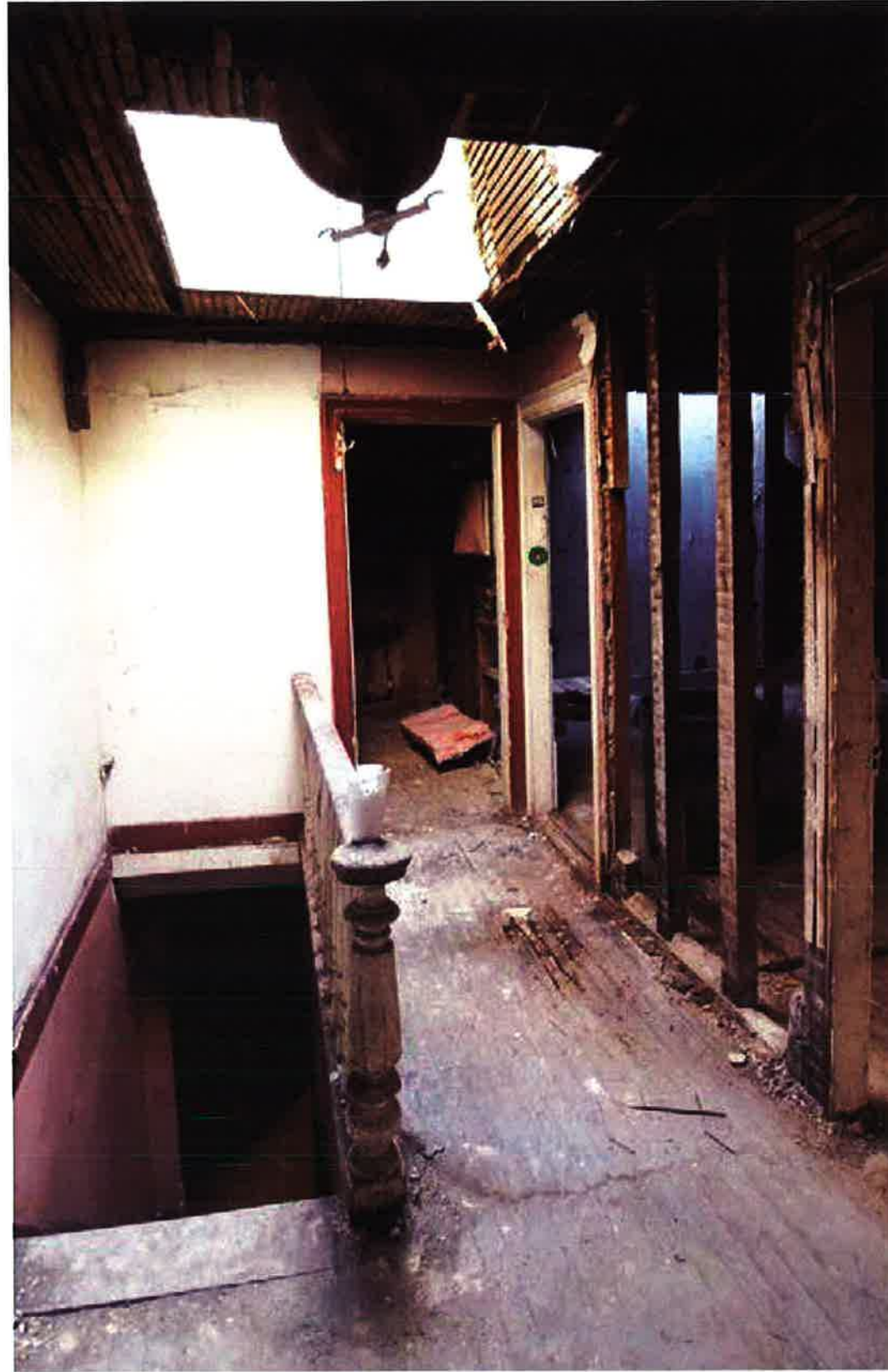
EXISTING CONDITION - THIRD FLOOR 237 BLEECKER STREET
