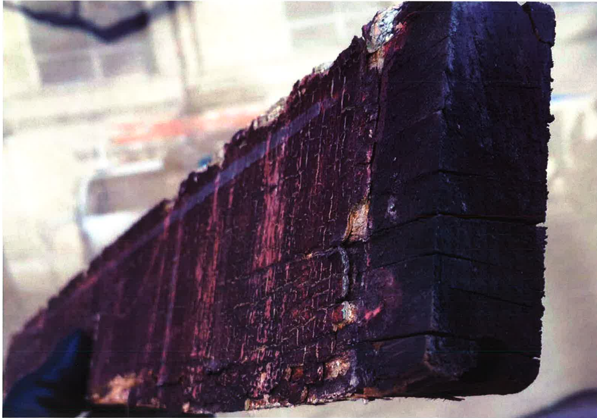
PAINTED WOOD SIDING WITH PAINTED MORTAR JOINTS 237 BLEECKER STREET
