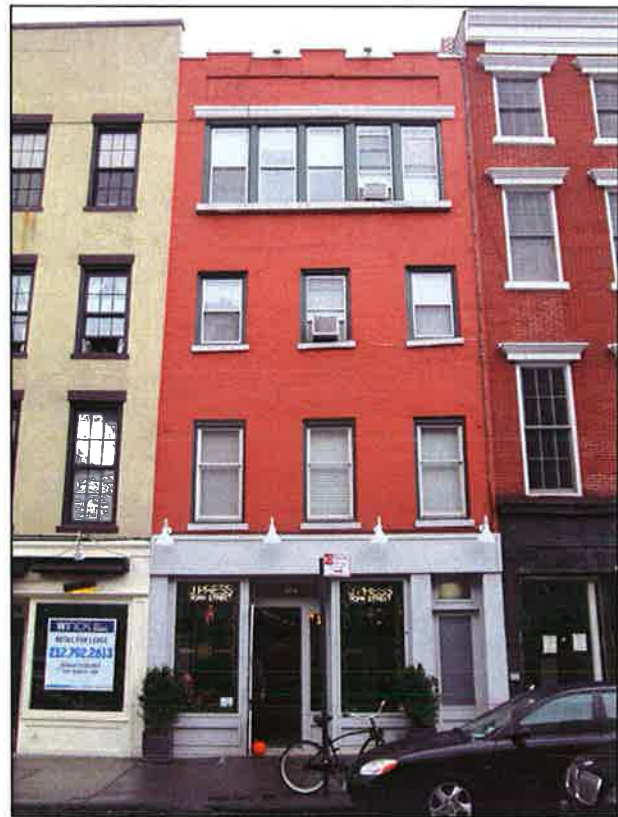
304 BLEECKER, EXISTING FACADE
