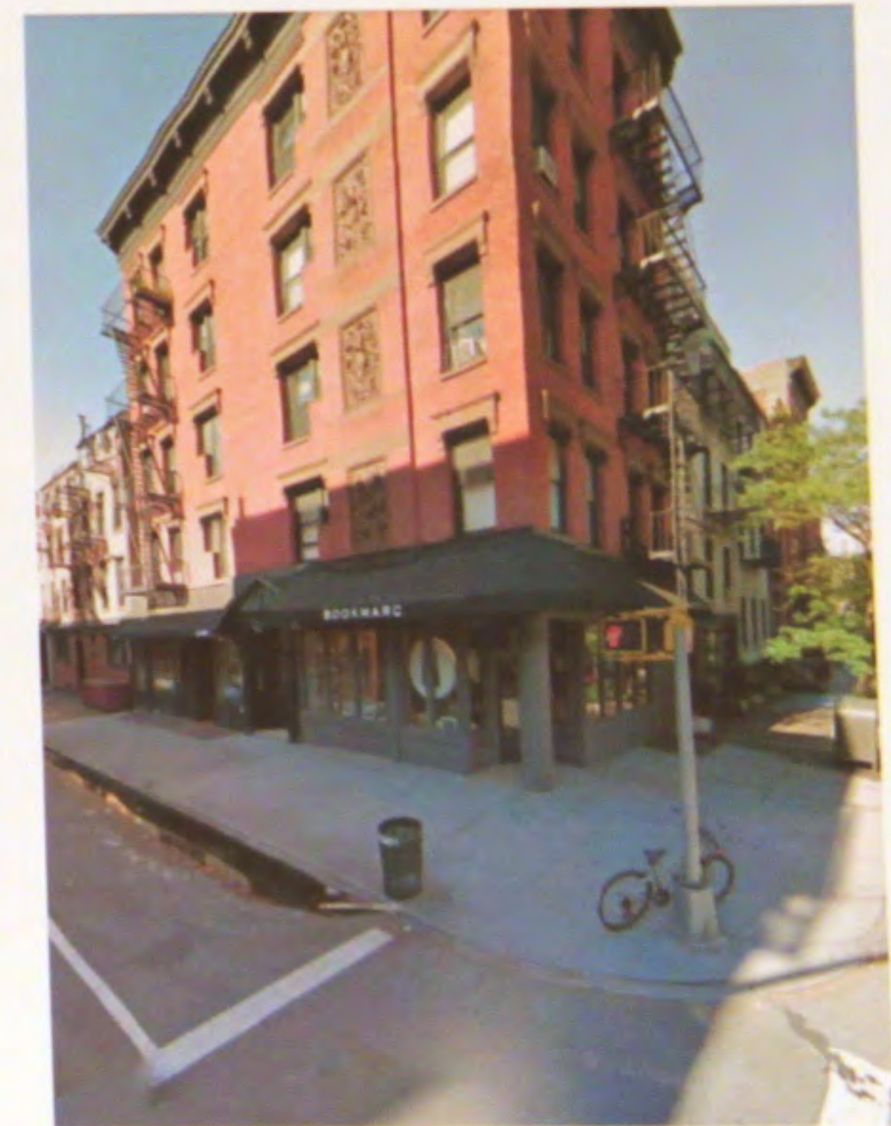
EXISTING CORNER PHOTO
