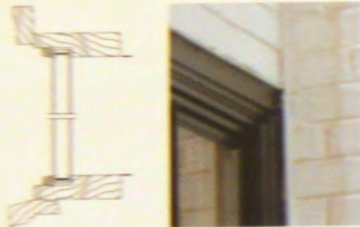
STOREFRONT FRAMING: CUSTOM WOOD FIXED FRAMING
