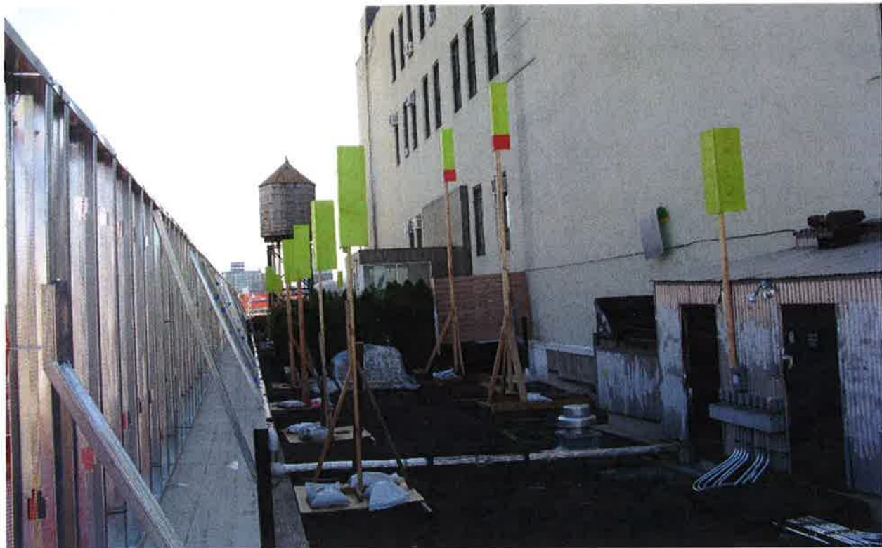
Mock-up Marker Posts installed on East Side of Main Roof
