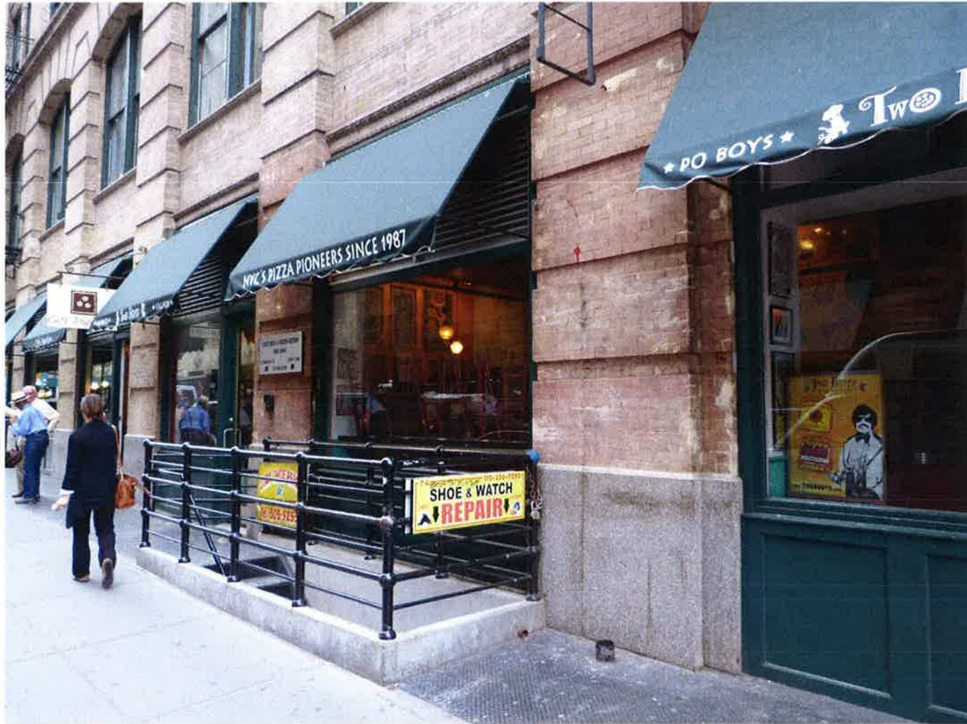
New Restorative Storefront on West Side of Bleecker St.
