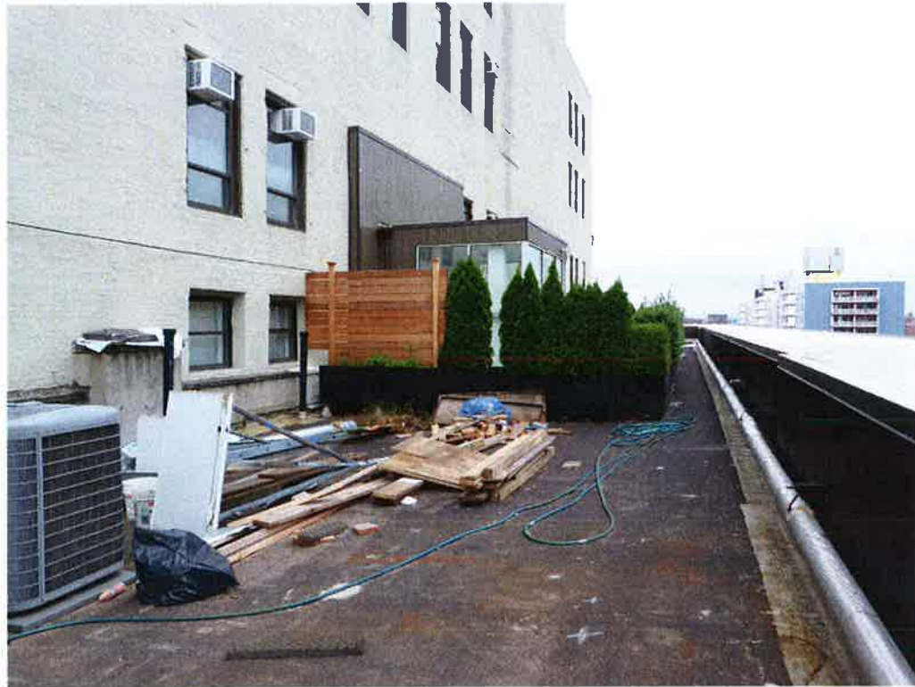
View of Roof Looking West
