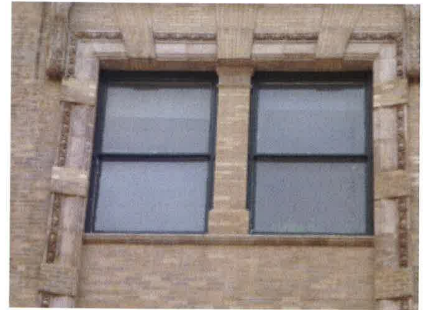
TYPICAL WINDOW - EXISTING CONIDITIONS
