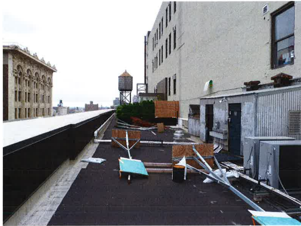
View of Roof Looking East
