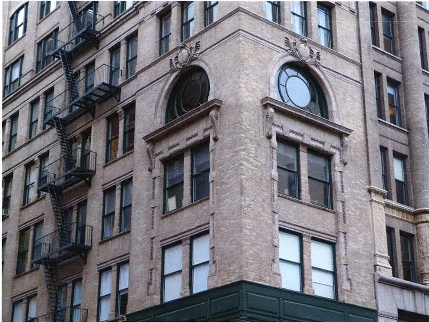
Cleaned and Repointed Masonry at Broadway and Bleecker Street
