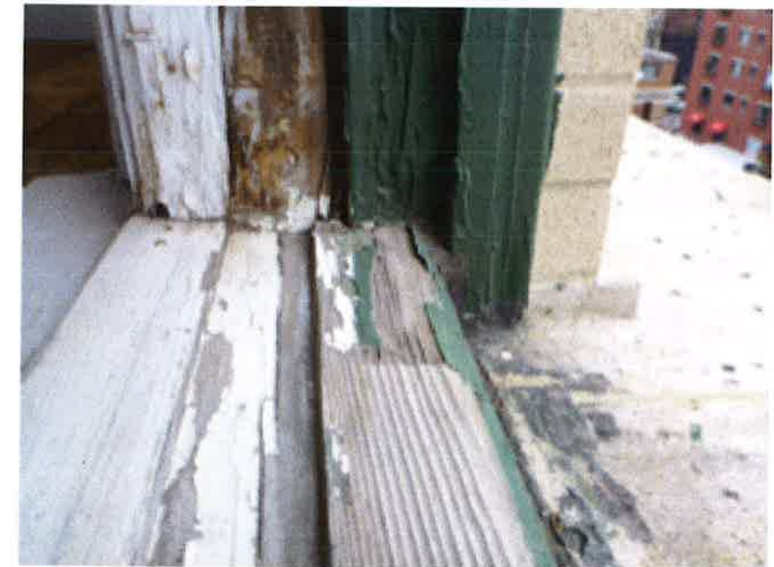
TYPICAL WINDOW - EXISTING CONIDITIONS
