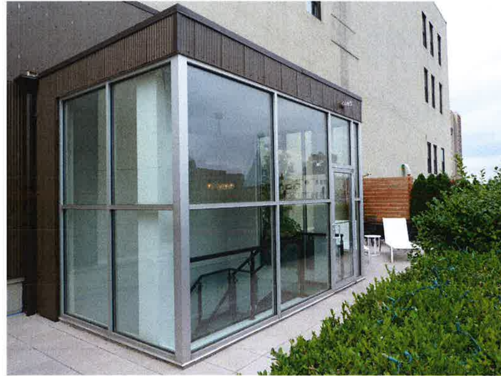
Private Deck and Stair Bulkhead
