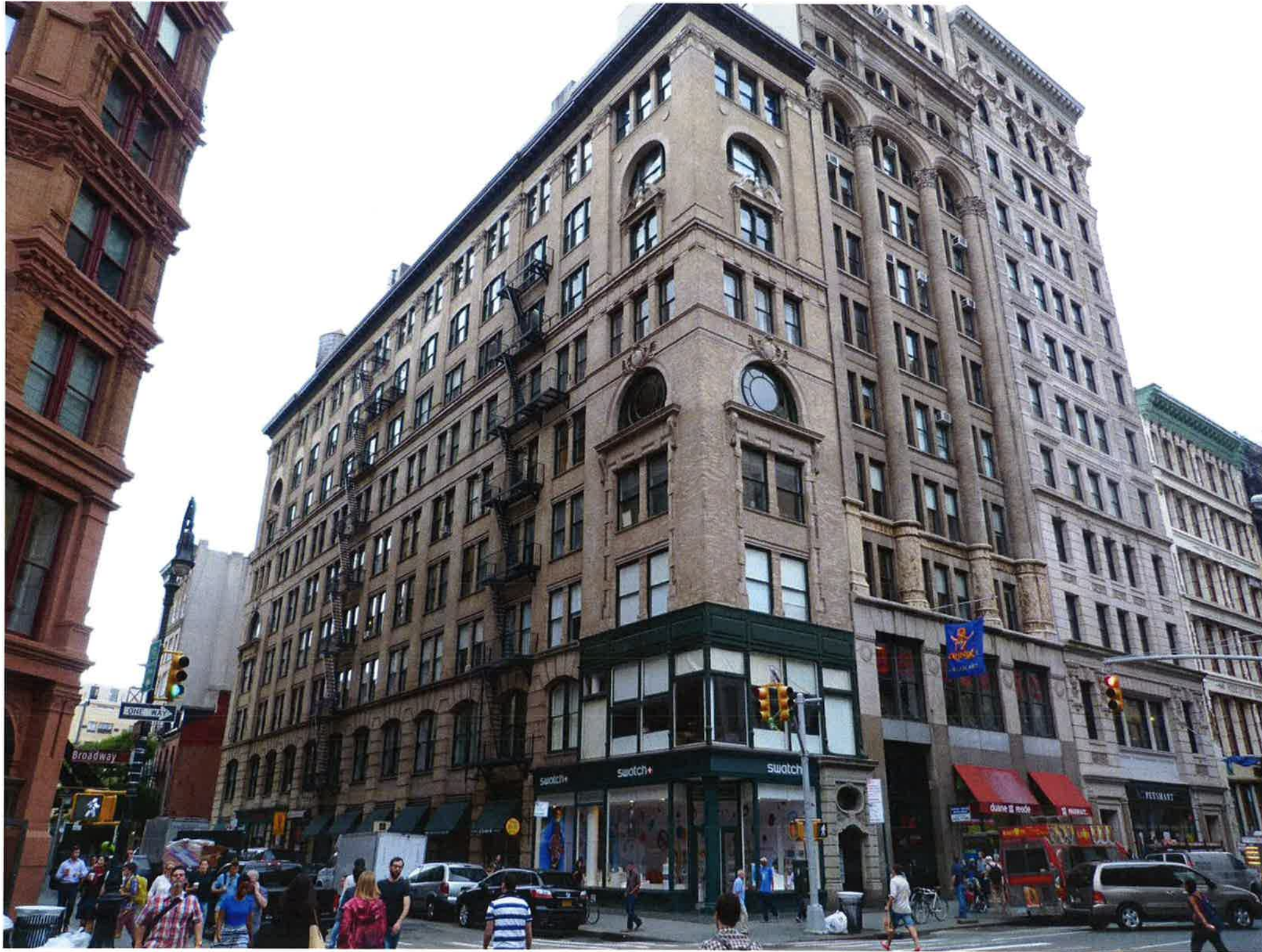
Present Condition, View Southeast
