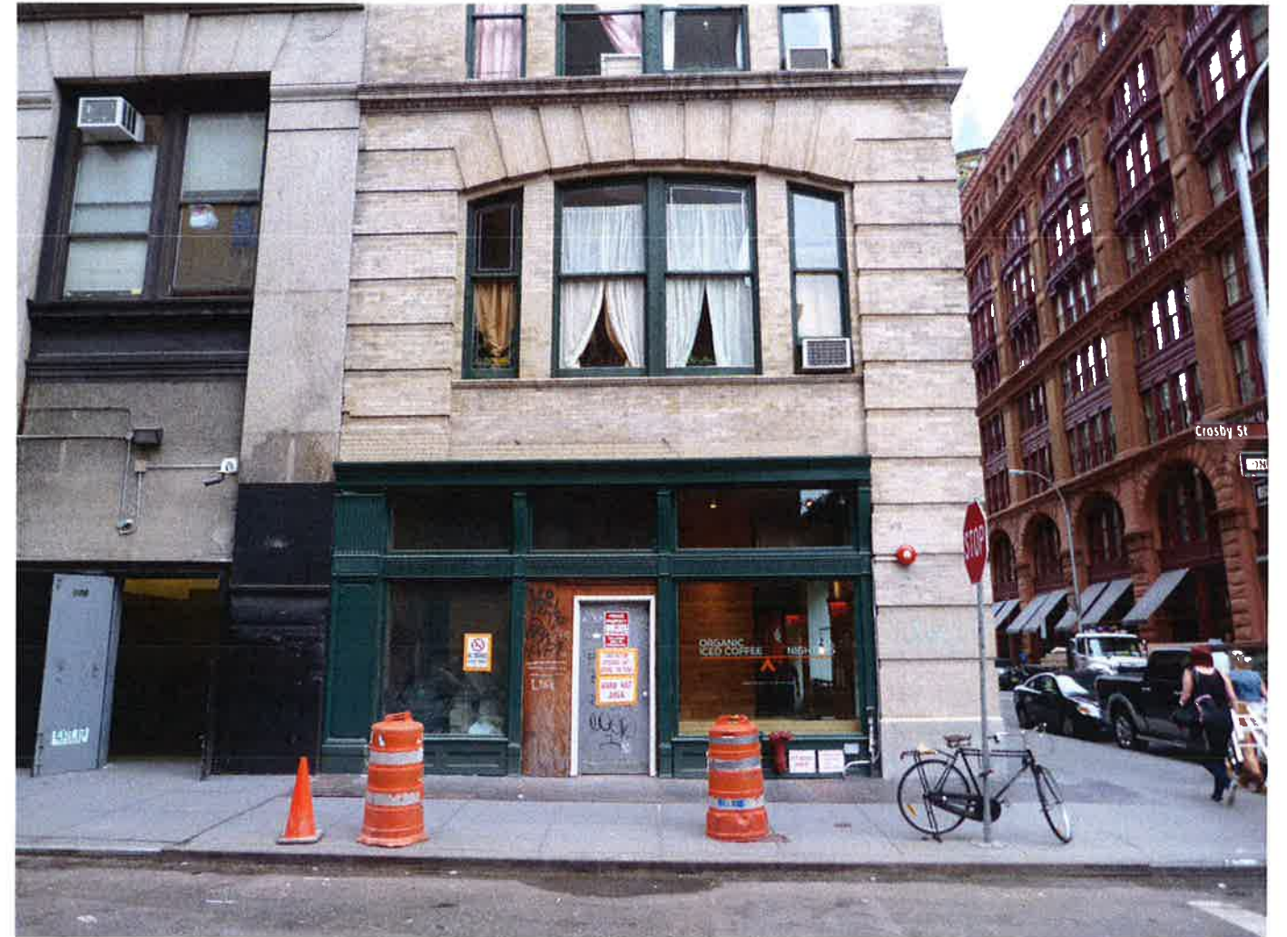
Storefront Repairs in Progress on Crosby St.
