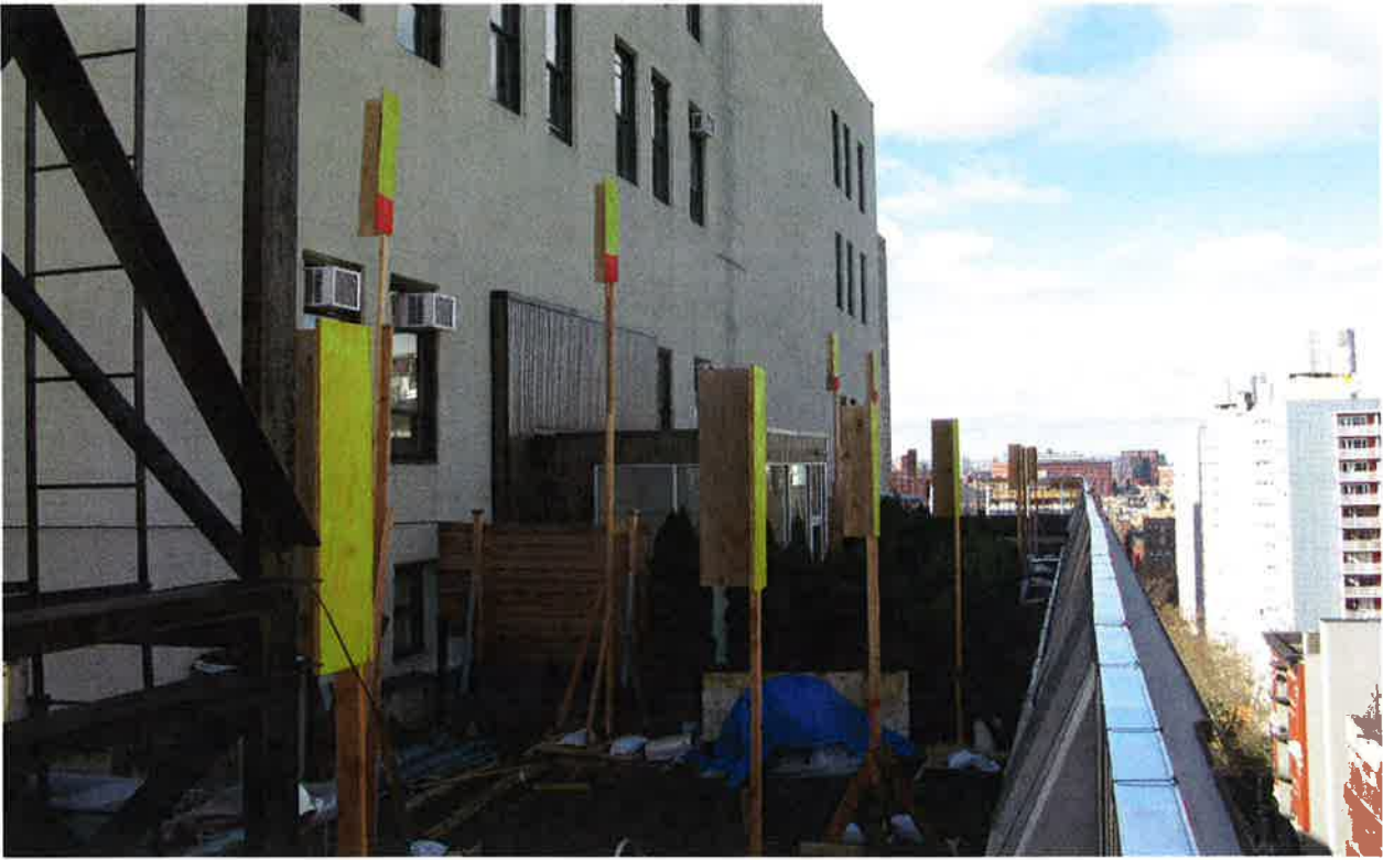
Mock-up Marker Posts installed on West Side of Main Roof
