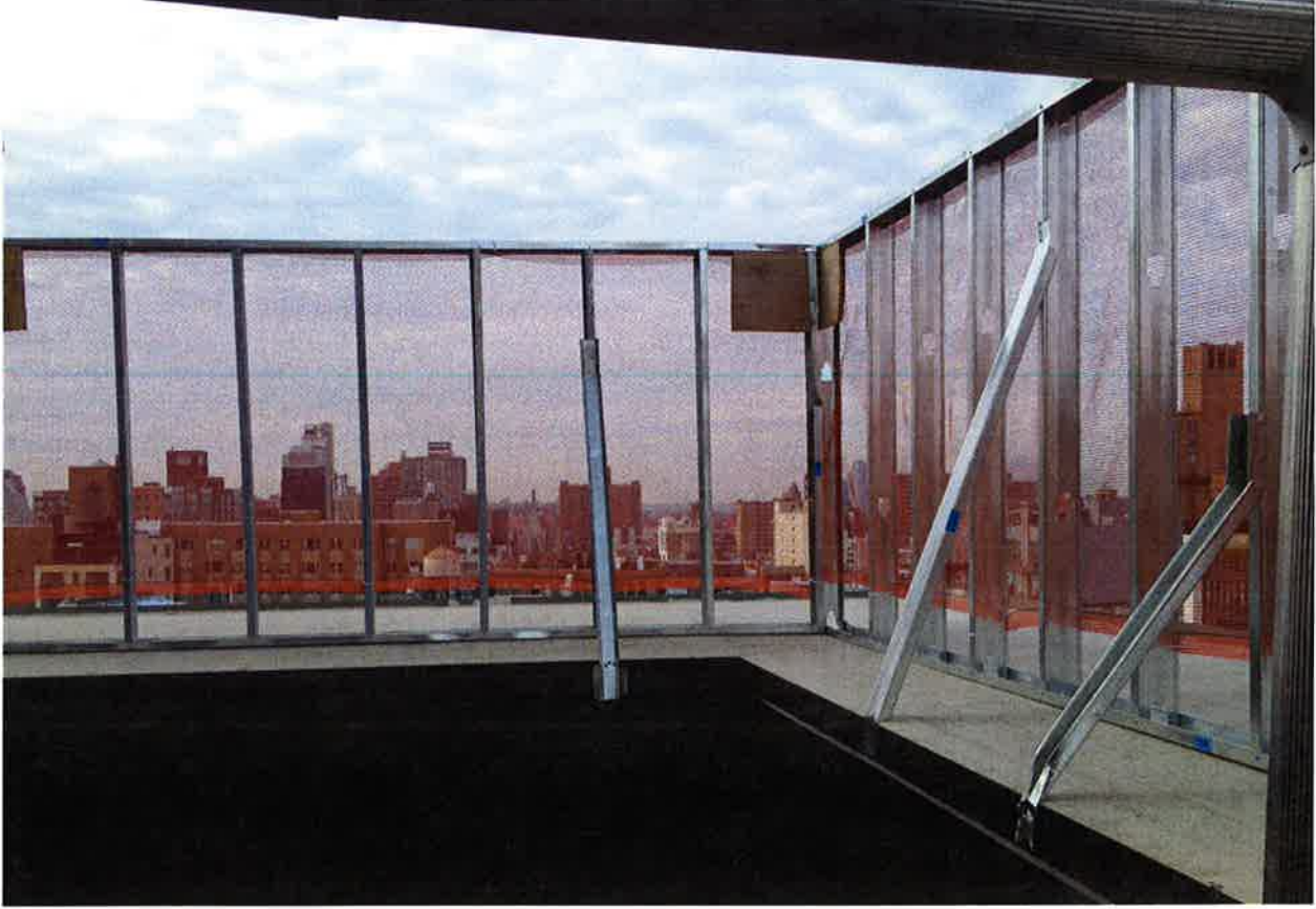
Mock-up of Balustrade installed on North and West Roof Parapet
