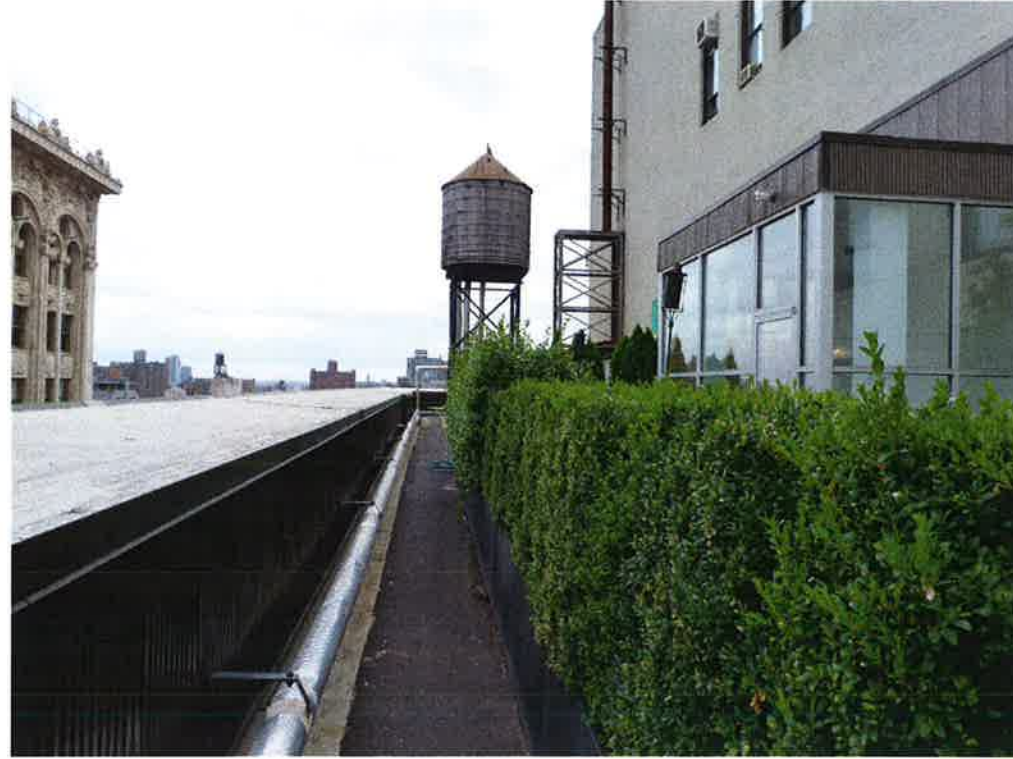
Private Deck and Garden at Center of Roof, Looking East
