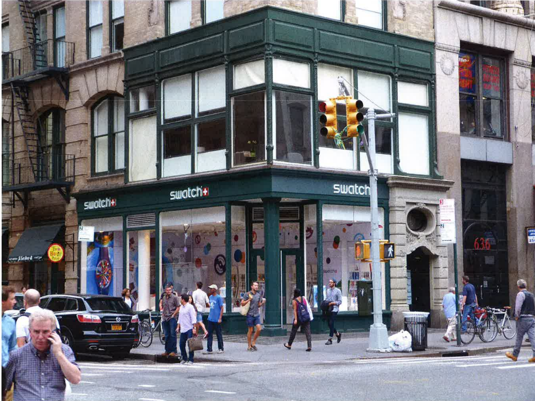
Repaired two-story Corner Storefront at Broadway and Bleecker Street
