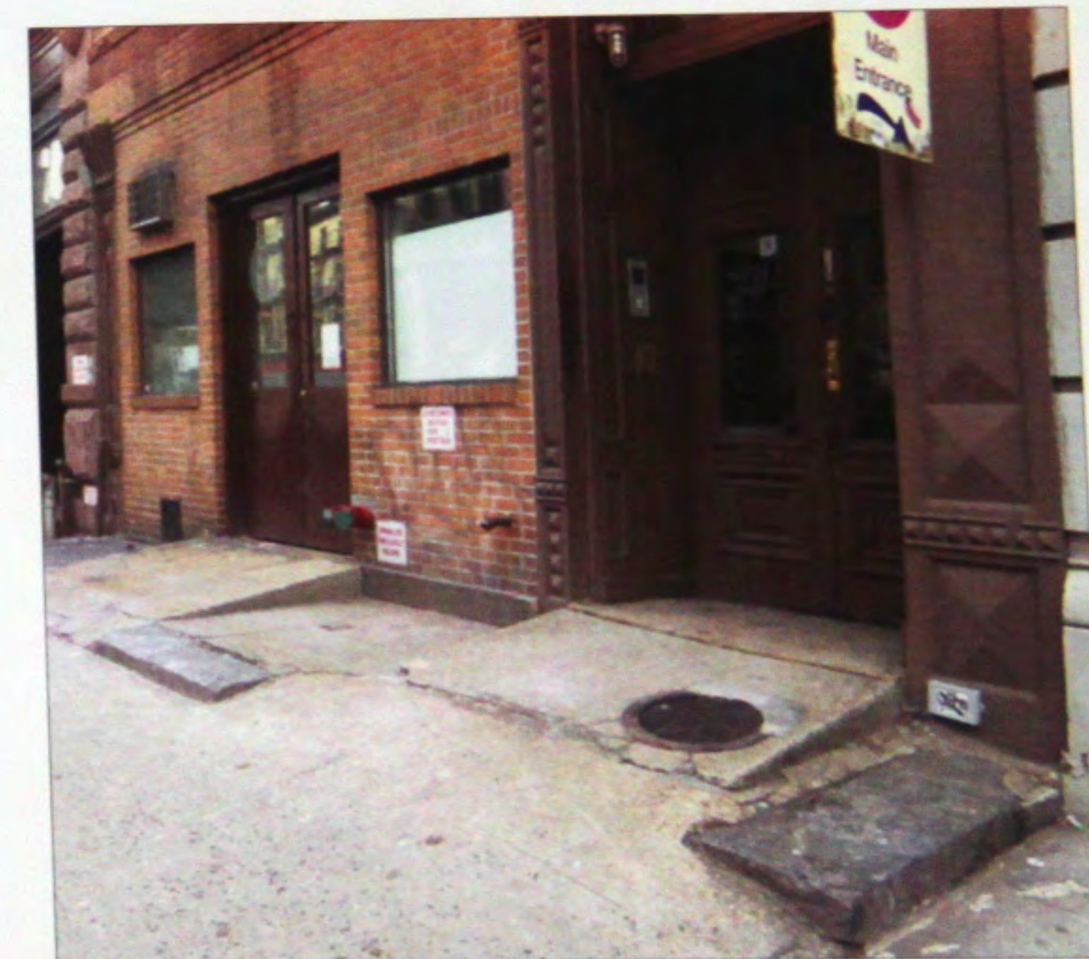
EXISTING STOREFRONT DETAIL & SIDEWALK CONDITION
