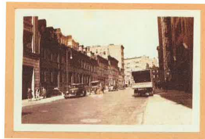
PICTURED ABOVE: HISTORIC PHOTOS SHOWING VARIOUS LIGHT AND DARK WINDOWS ON VANDAM STREET.
