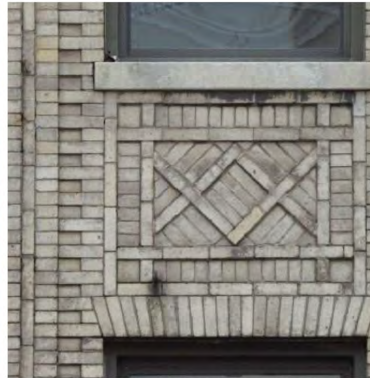
410 WEST 14TH STREET - BRICK FRAME AND SPANDREL
