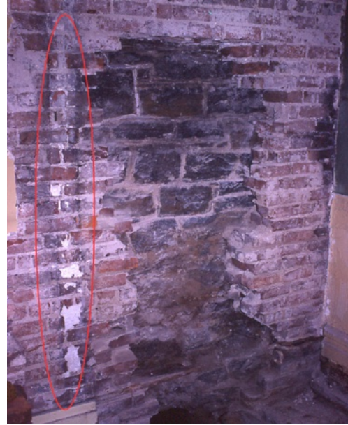
Left: 1936 blueprint showing “partition removed.” The location of the passageway is marked in yellow. Right: 1974 photograph showing mark consistent with location of the partition.
