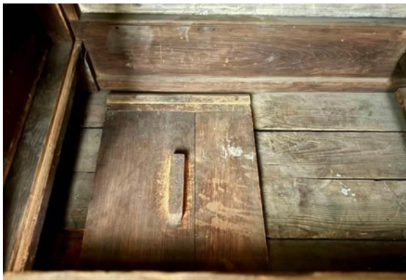
Photo 2. Left: Lifting the handle provides access to the passageway, approximately 2' x 2'. Right: After entry, the handle closed the hatch from inside. Note the candle wax drippings left by those traversing the passageway.
