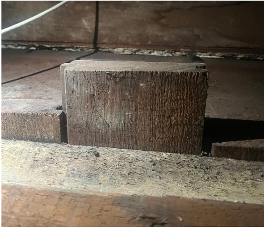
Above: Photo 5. The base of the passageway has no floorboards. Parlor level floorboards adjacent to the passageway are of uneven lengths, as pictured, indicating they were not cut away at a later date.
