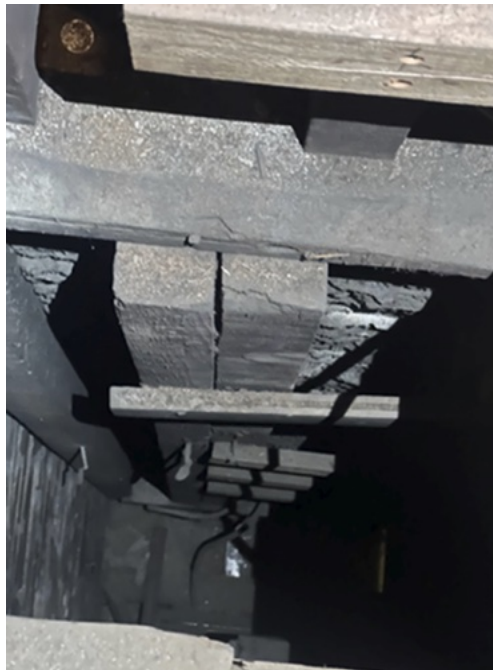
Above: Photo 4. The passageway has a built-in ladder from the 2nd floor (bedroom) level down to the 1st floor (parlor) level
