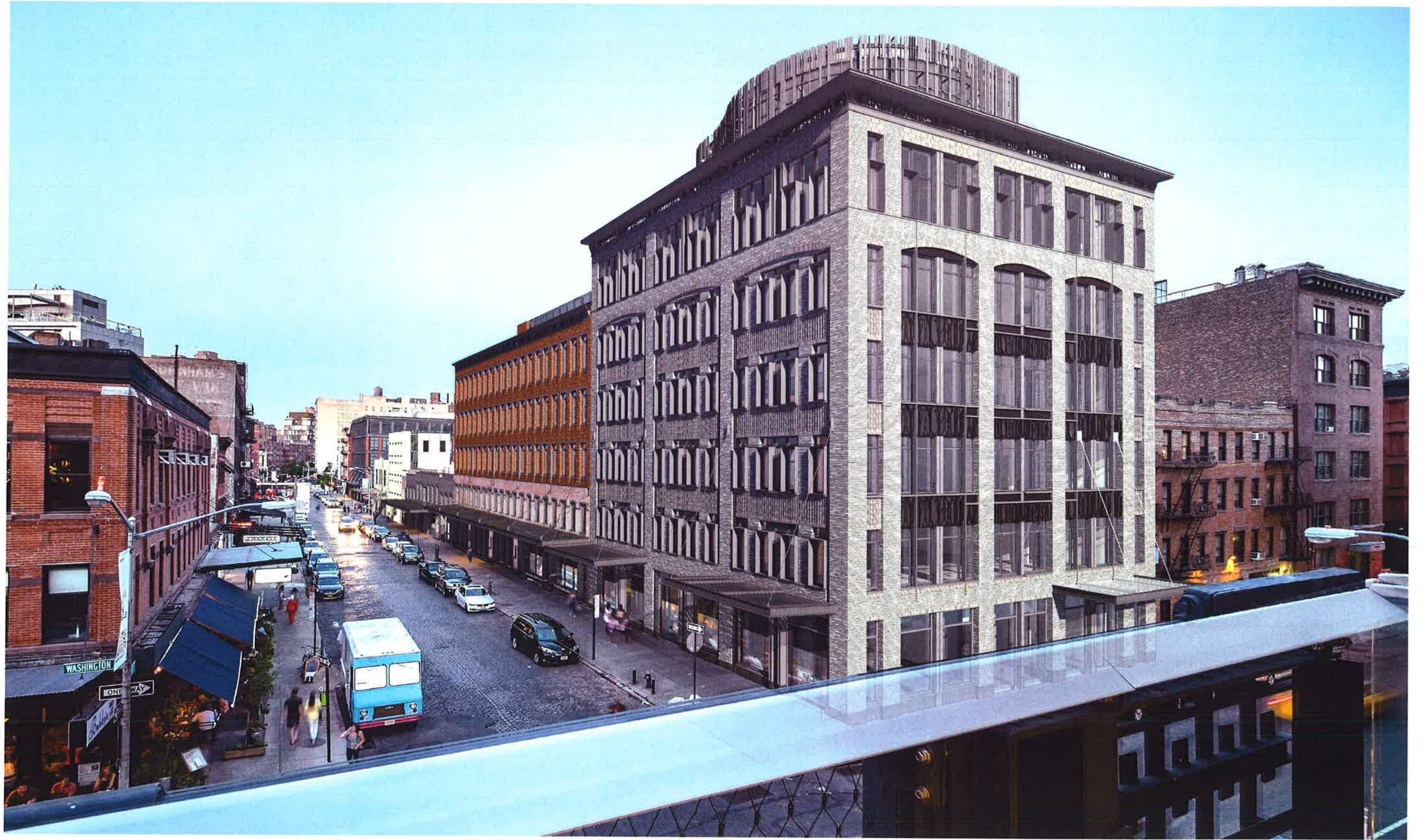
VIEW FROM HIGH LINE 46-74 GANSEVOORT STREET
