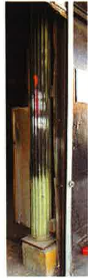
CAST IRON COLUMNS BEHIND EXISTING INFILL
