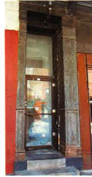
CAST IRON COLUMNS BEHIND EXISTING INFILL
