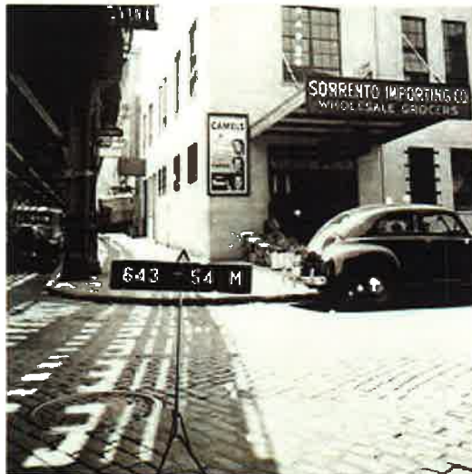
SHADOW UNDER HISTORIC ELEVATED RAIL
