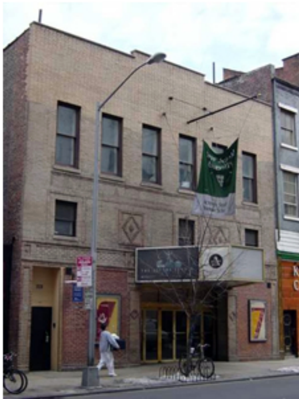
Circle in the Square Theater before demolition, as requested for landmark status by GVSHP.
