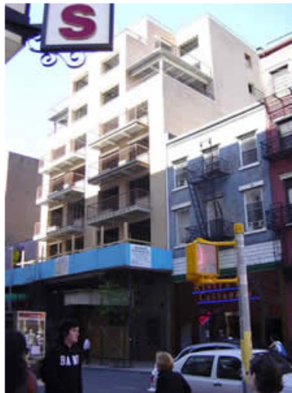
Circle in the Square site post-demolition.
