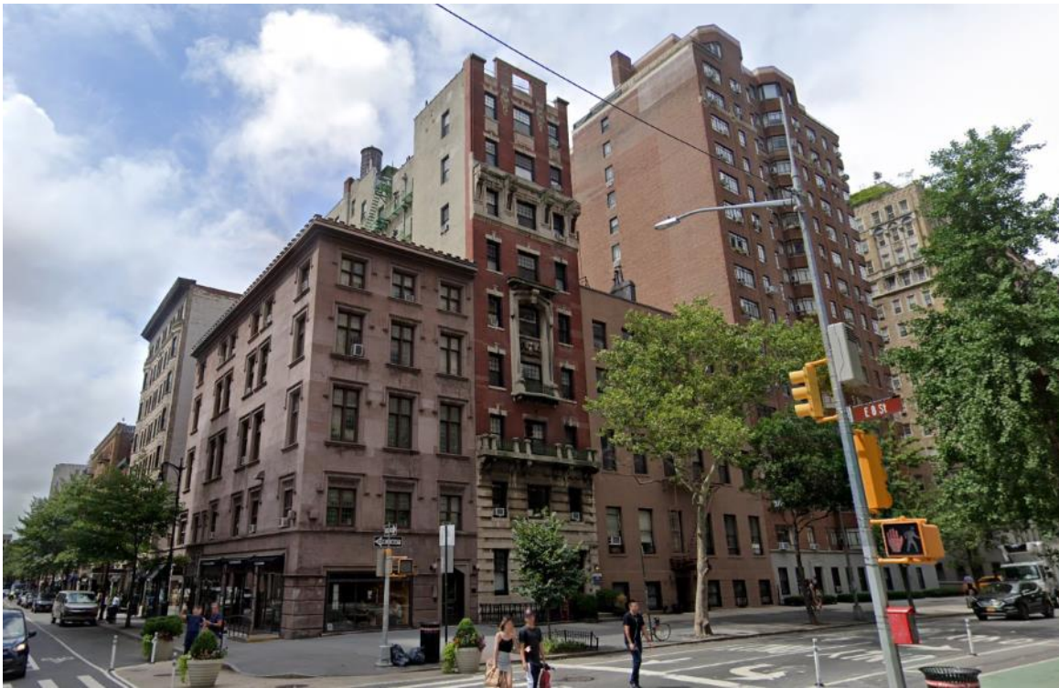
14-16 Fifth Avenue is the 5-story building in the center of the block.
